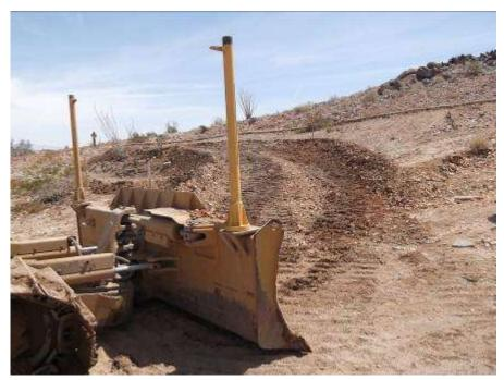
**Figure 6.** Grading activities initiated prior to topsoil salvage at Tower 2518. The blade mark is located within the area designated for salvage.
