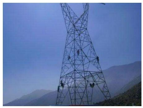
Figure 3. Tower assembly (crews backbolting) at Tower 1057.
