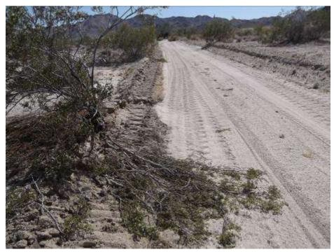
**Figure 7.** Heavy equipment tracks outside road limits between Towers 2433 and 2434 resulting in several crushed creosote bushes.
