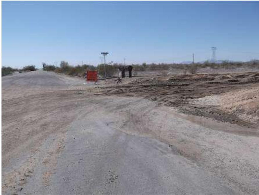
**Figure 7.** Excessive track-out identified at intersection of Chuckwalla and Corn Springs Roads.
