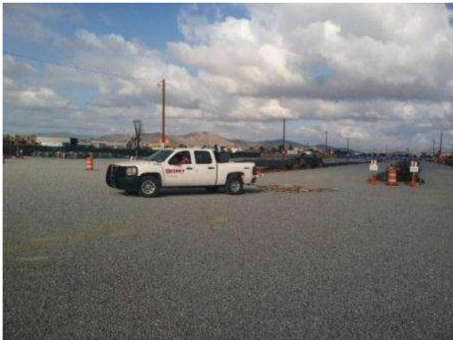
**Figure 10.** Contractor vehicle dragging a piece of fencing to comb gravel within the Meniffee Yard.
