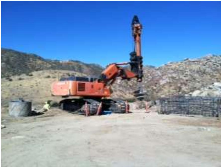
**Figure 3.** Foundation drilling activities at Tower 1071.
