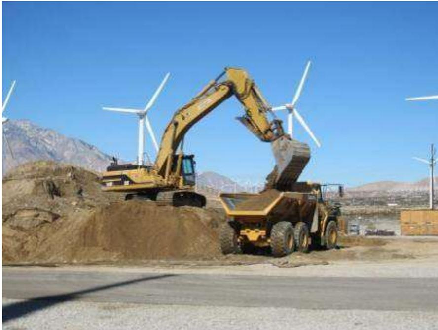
**Figure 10.** Stockpiled soil being transported from within the existing Devers Substation to the expansion area.
