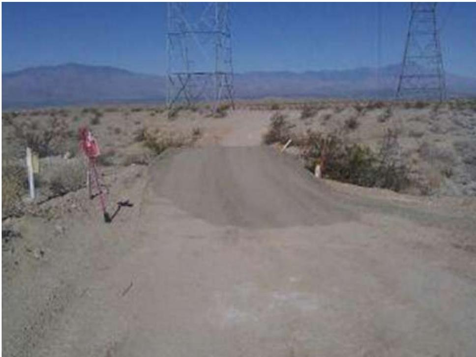
**Figure 4.** Gravel road base installed along an unapproved road near Tower 2303.
