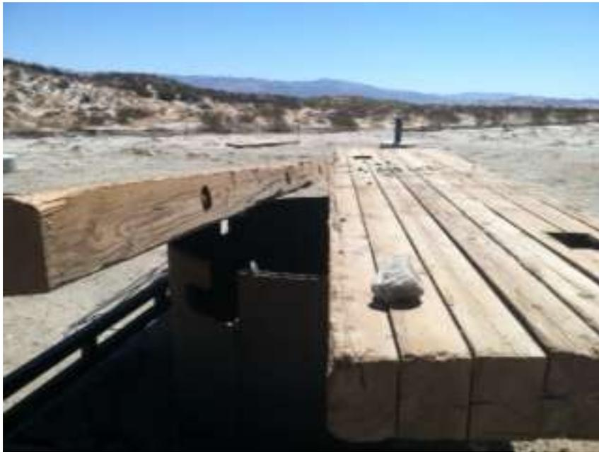
**Figure 5.** Inadequately covered foundation excavation at Tower 2015.
