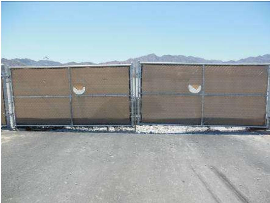
**Figure 10.** Substantial gap underneath entrance gate at PAR Desert Center 2 Construction Yard.
