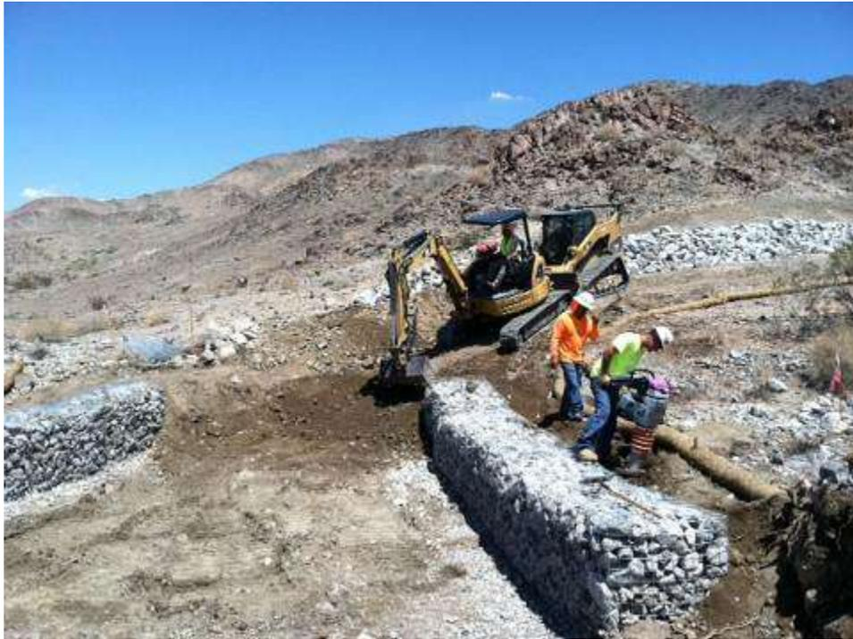
**Figure 1.** Wet crossing installation at Tower 2325.
