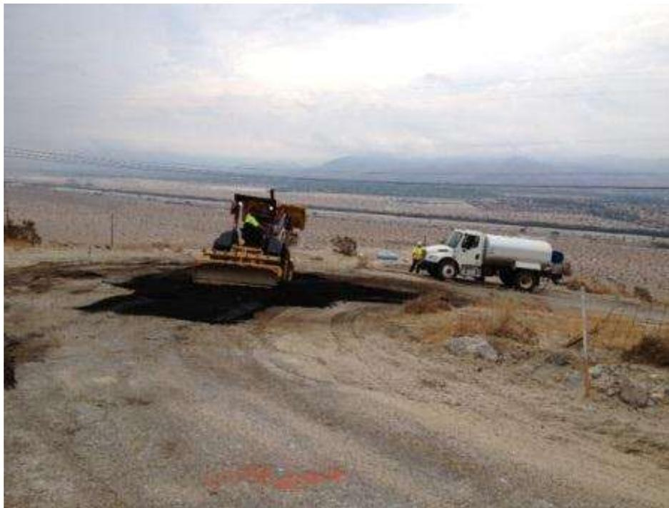
**Figure 2.** Asphalt repair on the access road to Tower 2117. (Photo Courtesy of FRED)
