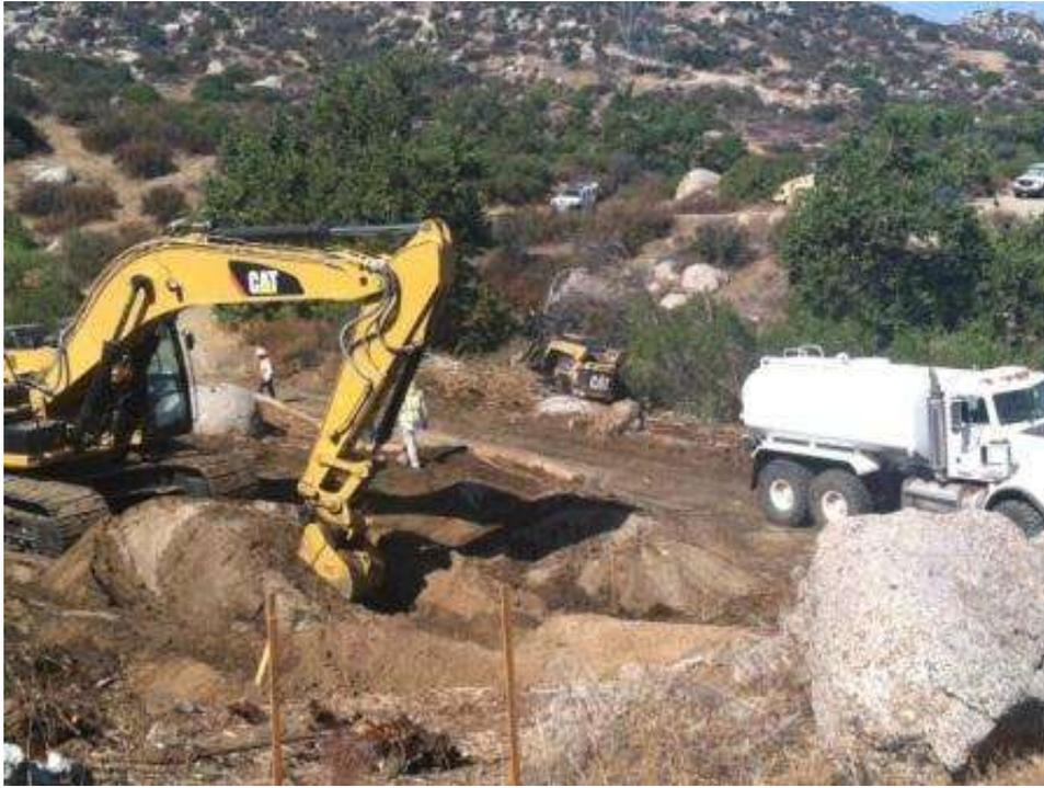
**Figure 3.** Excavation for the installation of the crane pad at Tower 1140.
