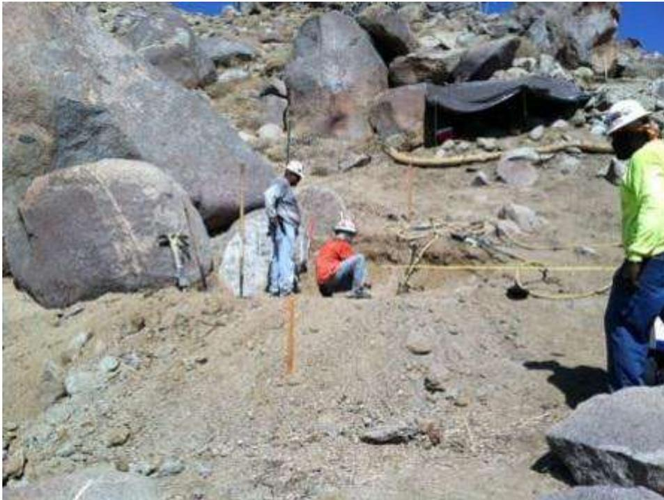
**Figure 4.** Rock clearing at tower foundation preparation at Tower 1032.
