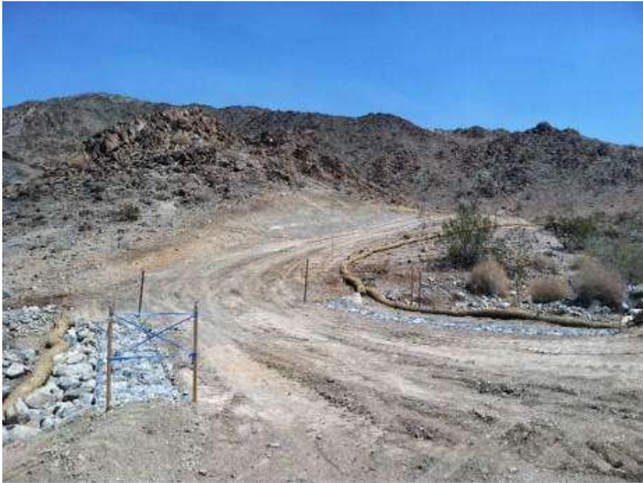
**Figure 1.** Wet crossing installation complete at Tower 2325.
