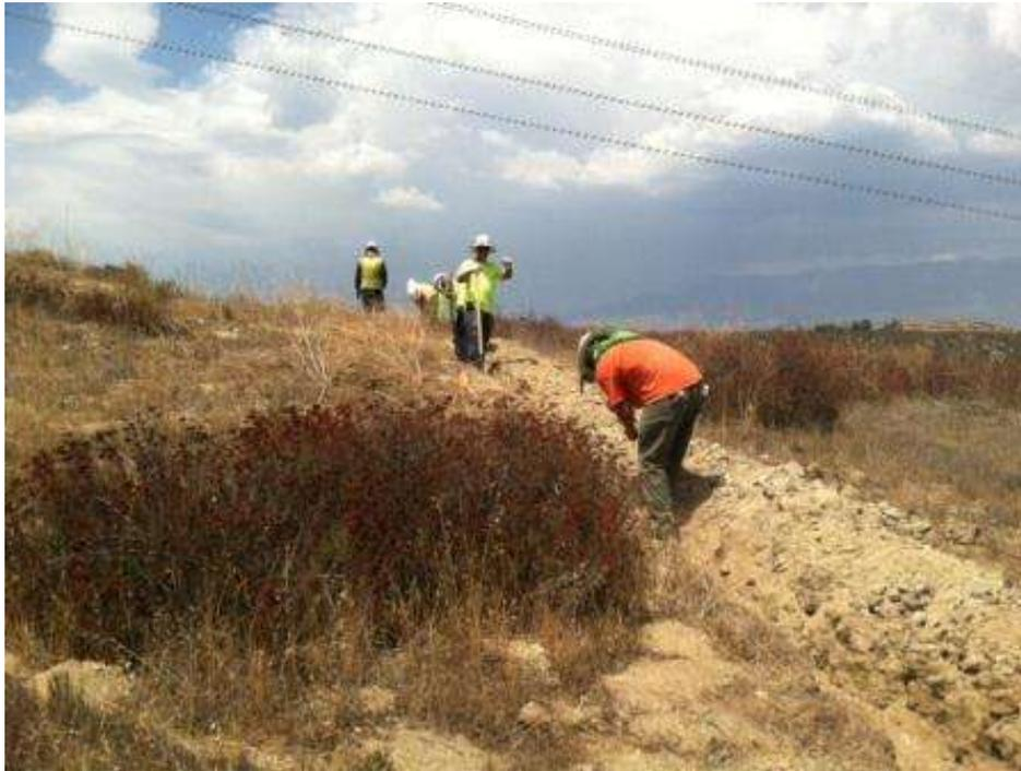
**Figure 5.** Trenching for the installation of the Stephen's kangaroo rat exclusionary fencing at Tower 1100.
