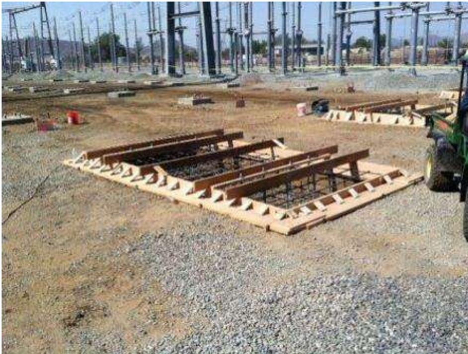
**Figure 10.** Preparation for concrete pouring for a foundation within the Valley Substation.
