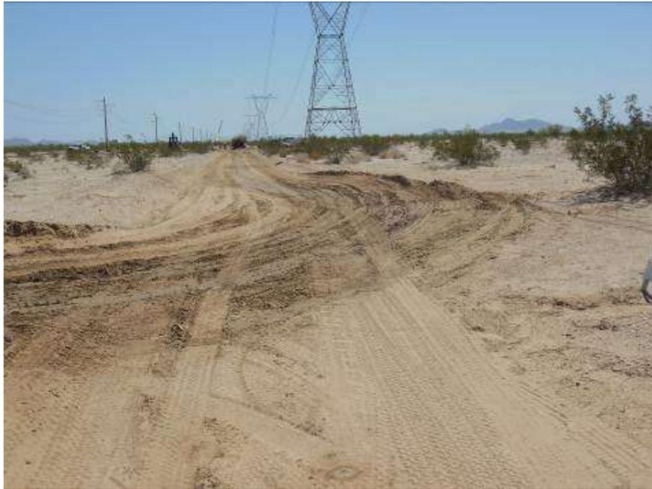
**Figure 7.** Multiple vehicle/equipment tracks observed outside of the approved road limits between Towers 2618 and 2619.
