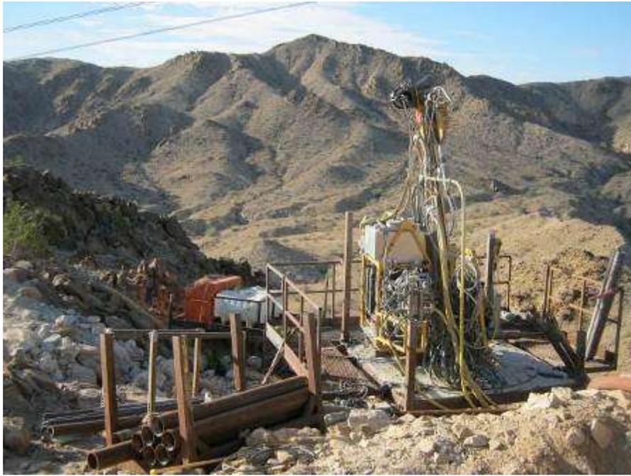
**Figure 3.** Micropile drilling at Tower 2424.
