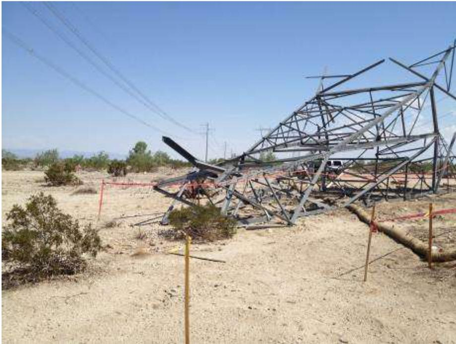
**Figure 8.** Tower section that had fallen over due to inclement weather and partially landed outside the disturbance limits at Tower 2538.
