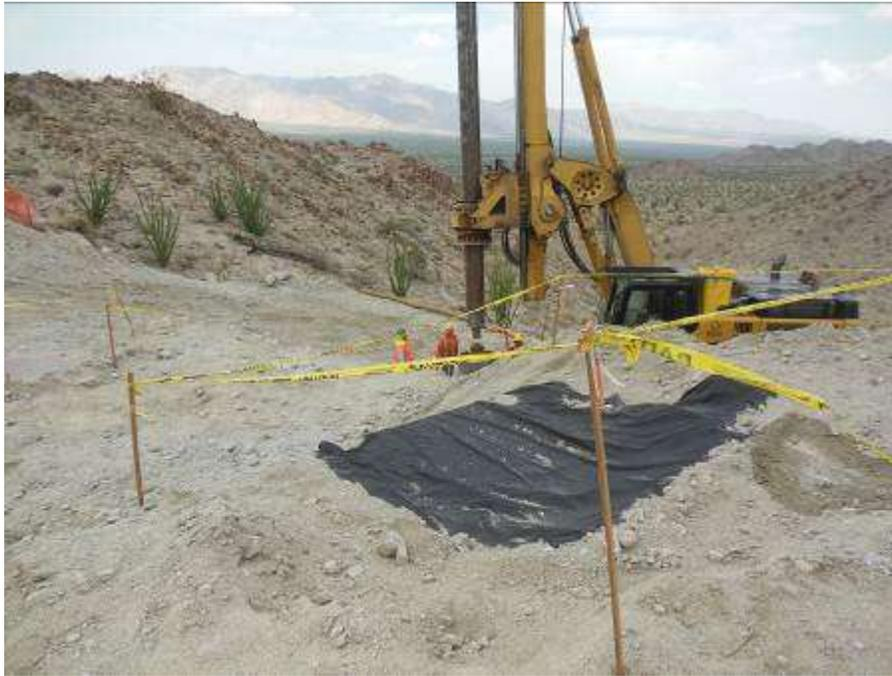
**Figure 7.** Properly covered foundation excavation at Tower 2547.
