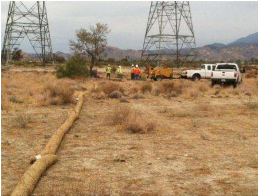
**Figure 5.** Installation of BMPs at DV Pullsite R2 adjacent to Towers 1062 and R2.
