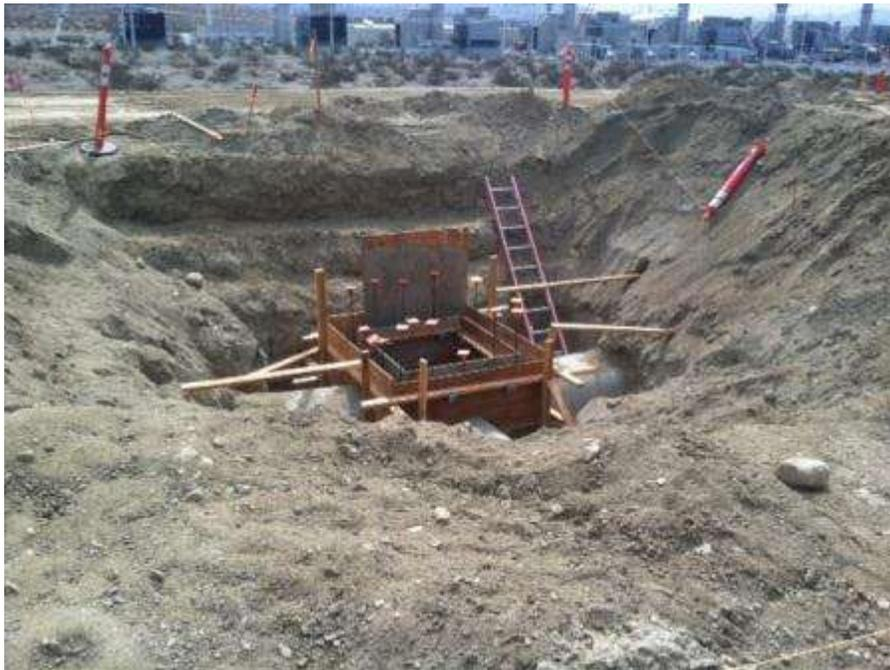
**Figure 10.** Wooden forms for a manhole over the newly installed waterline within the Devers Substation Expansion area.
