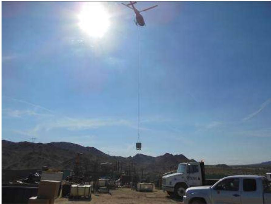
Figure 3. Transfer of grout from hopper to bucket at HLZ H5 for micropile activities at Tower 2424.
