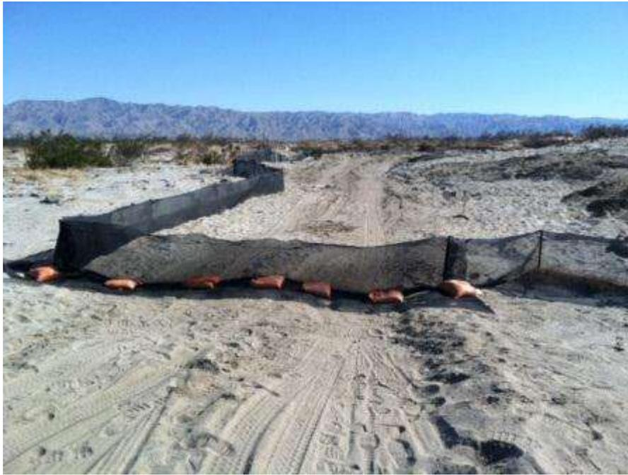
Figure 5. Repairs to Coachella Valley Fringe-toed Lizard exclusionary fencing completed at Tower 2013.
