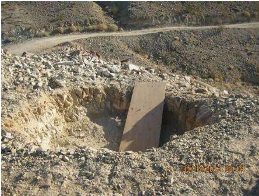
Figure 9. Wildlife ramp to prevent entrapment at Tower 2310X.
