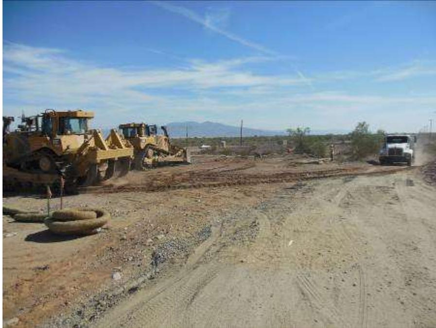
Figure 1. Grading activities at Guard Structure RB-GS06.
