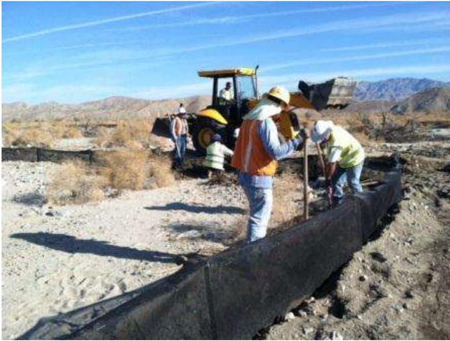
Figure 3. Installation of Coachella Valley Fringe-toed Lizard exclusionary fence at Wire Site 14/ Pull Site 15.
