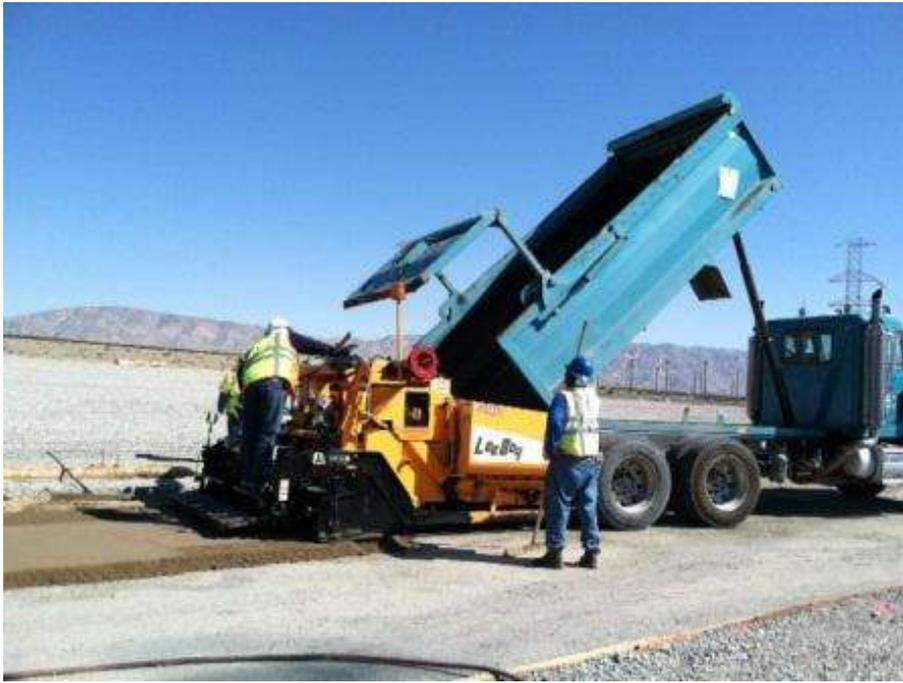
Figure 9. Installation of natural pavement at the Devers Substation.
