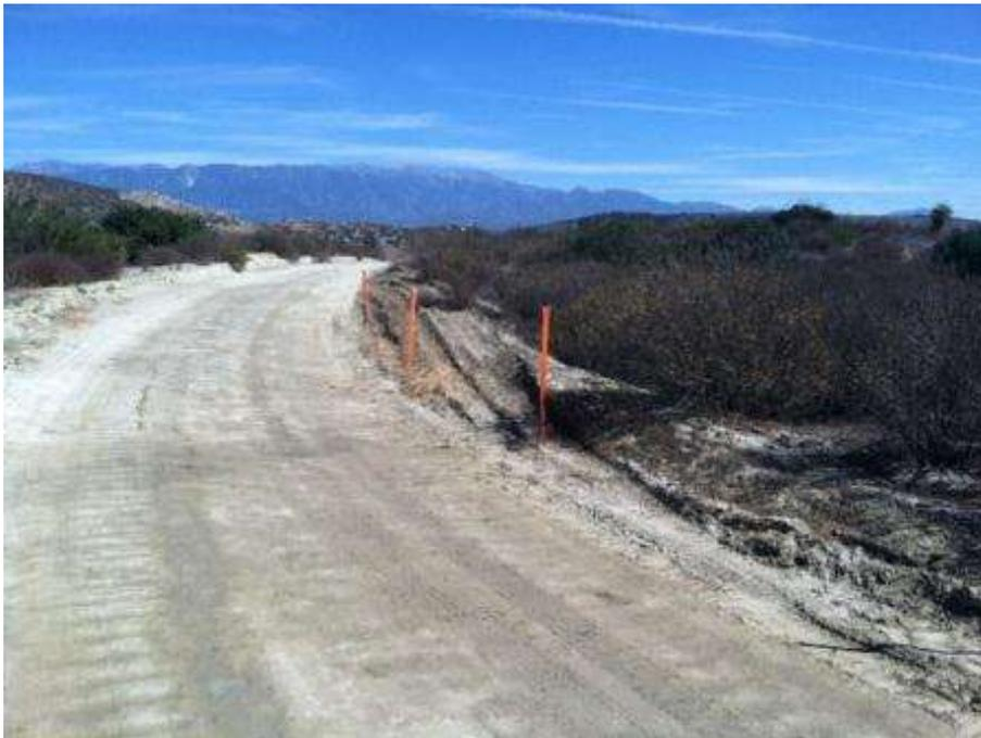
Figure 4. Tire tracks observed outside of the approved access road boundaries near Tower 1105. Please note the stakes placed by the Biological Monitor and contractor Foreman to prevent future impacts.
