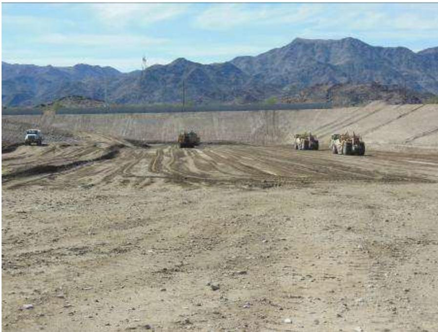
Figure 8. Backfilling of the drainage basin at Red Bluff Substation.
