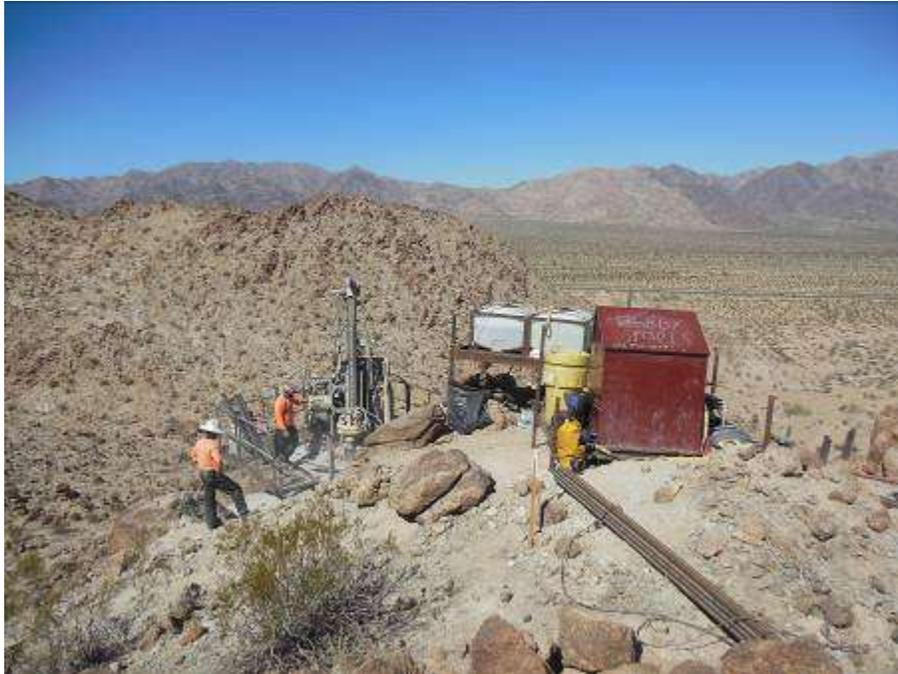
Figure 2. Micropile drilling at Tower 2422.
