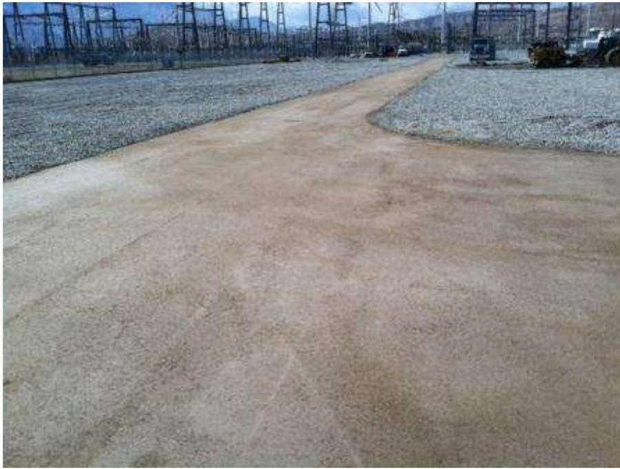
Figure 9. Curing Natural Pavement at the Devers Substation.
