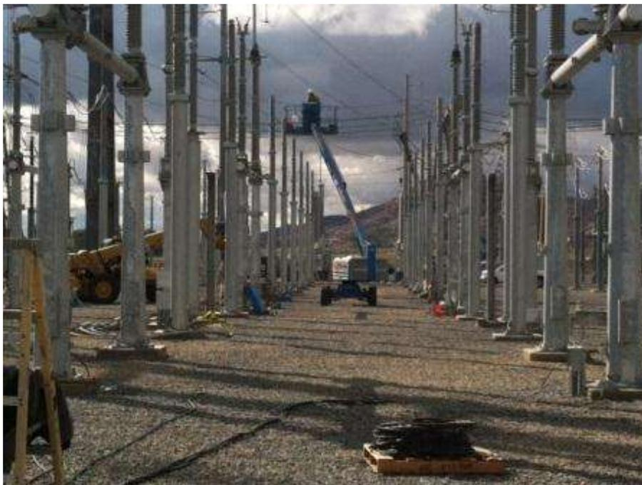
Figure 10. Erection of circuit breakers and disconnect switches at the Valley Substation.
