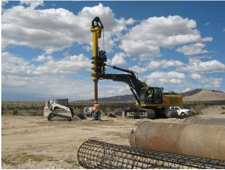
Figure 3. Foundation drilling at Tower 2306.
