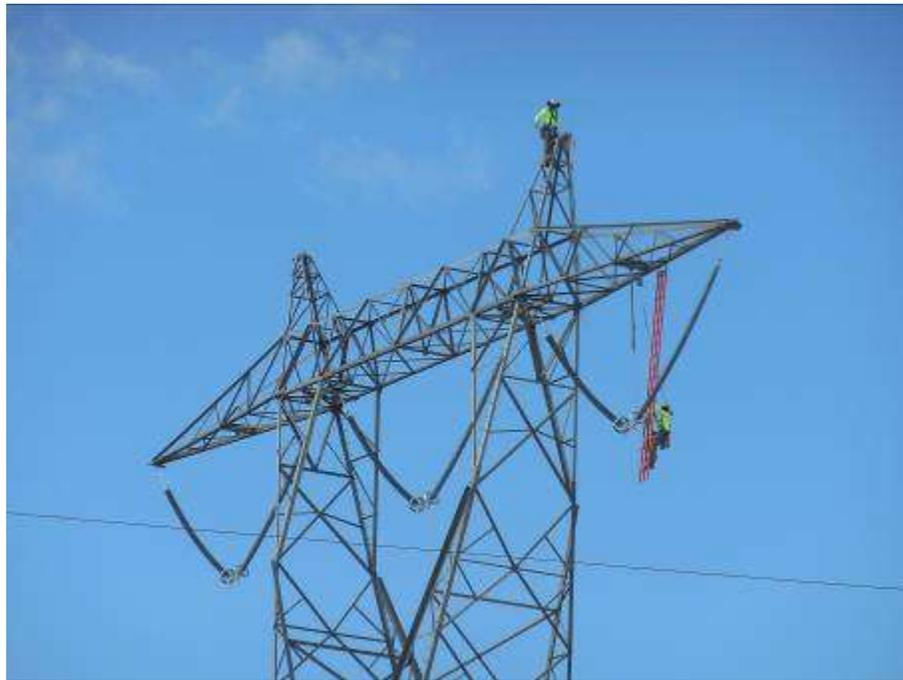
Figure 4. Installation of insulators at Tower 2543.
