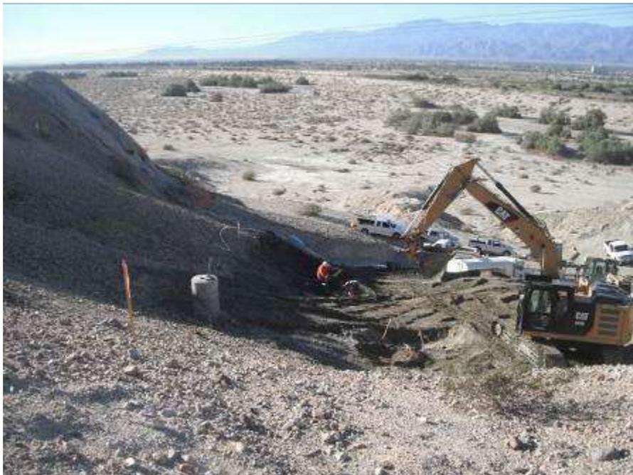
Figure 2. Site grading at Tower 2238. Photo courtesy of FRED.
