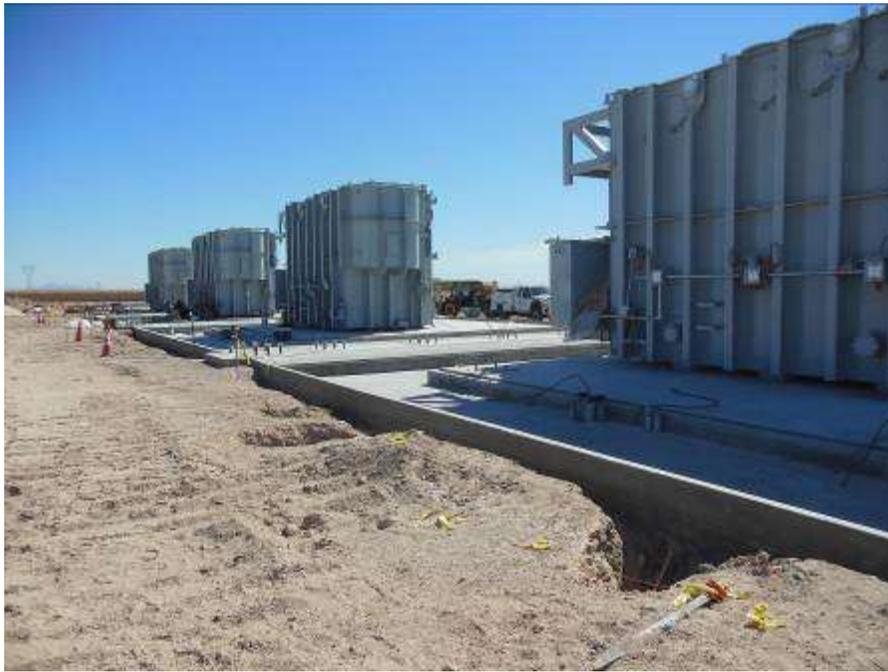
Figure 9. Transformers were relocated to the pad locations at CRS.
