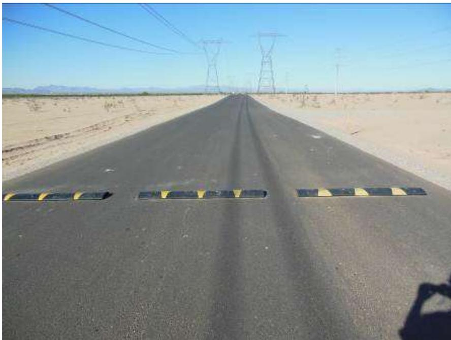
Figure 10. Temporary speed bumps installed along the CRS access road.
