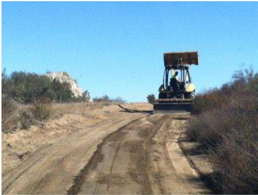
Figure 5. Maintenance grading of the ROW access road between Towers 1125 and 1131.
