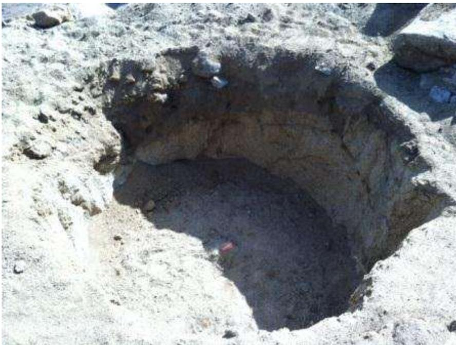
Figure 8. Uncovered steep-walled excavation at Tower 1036 that resulted in NCR #11.
