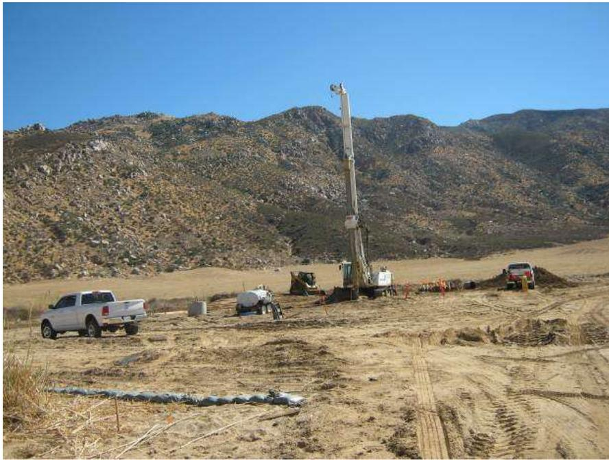
Figure 7. Foundation drilling at Tower 1084.
