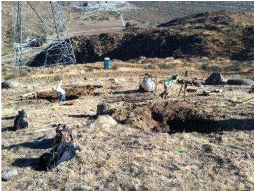
Figure 6. Micropile site preparation at Tower 1068.
