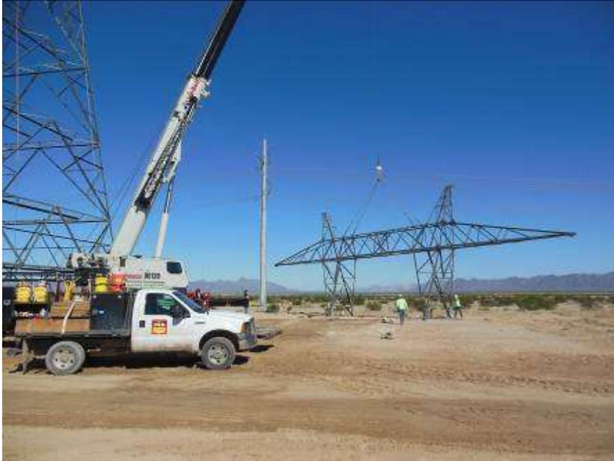
Figure 1. Preparing to install the bridge at Tower 2625.
