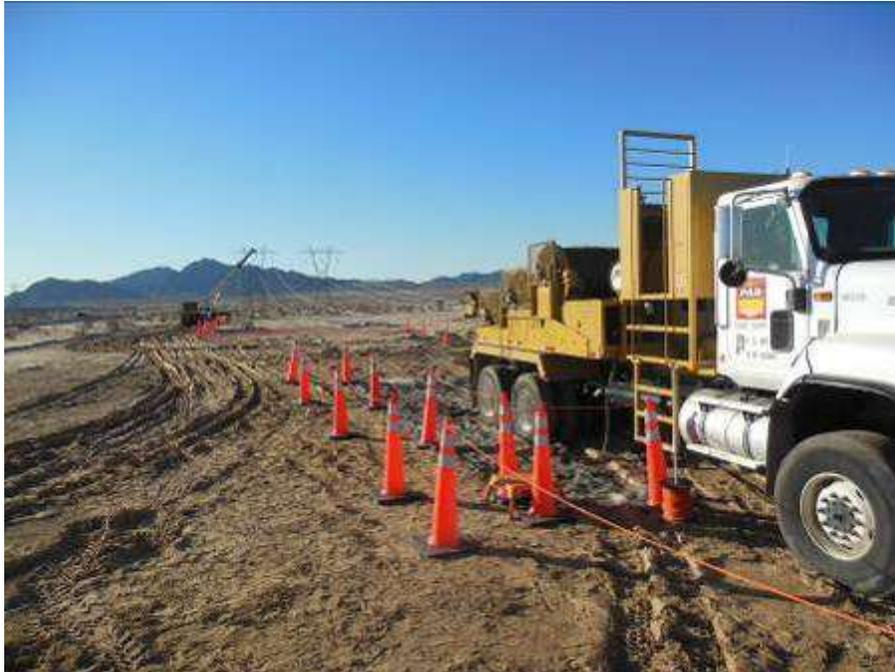
Figure 2. Stringing activities associated with the western CRS loop-in towers.
