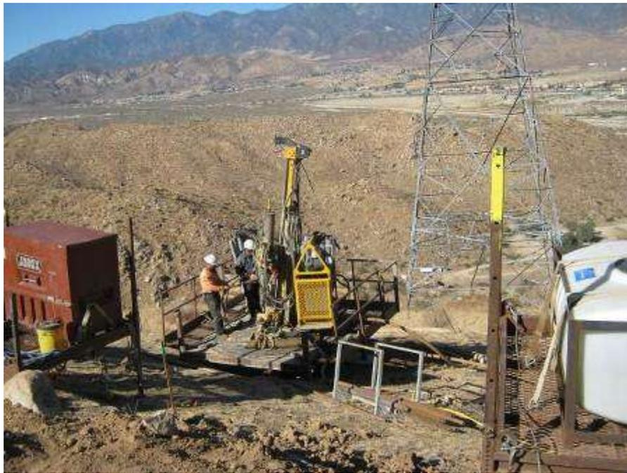
Figure 5. Micropile foundation drilling at Tower 1068.
