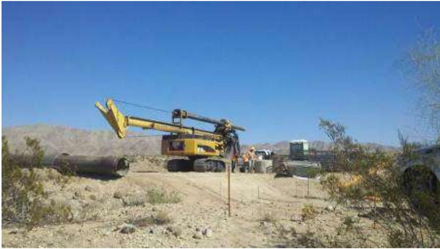
Figure 3. Foundation drilling at Tower 2265.
