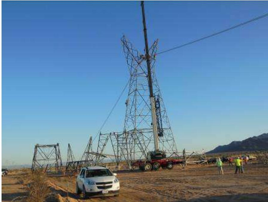
Figure 1. Wreck-out of existing DPV1 Tower M129-T1.
