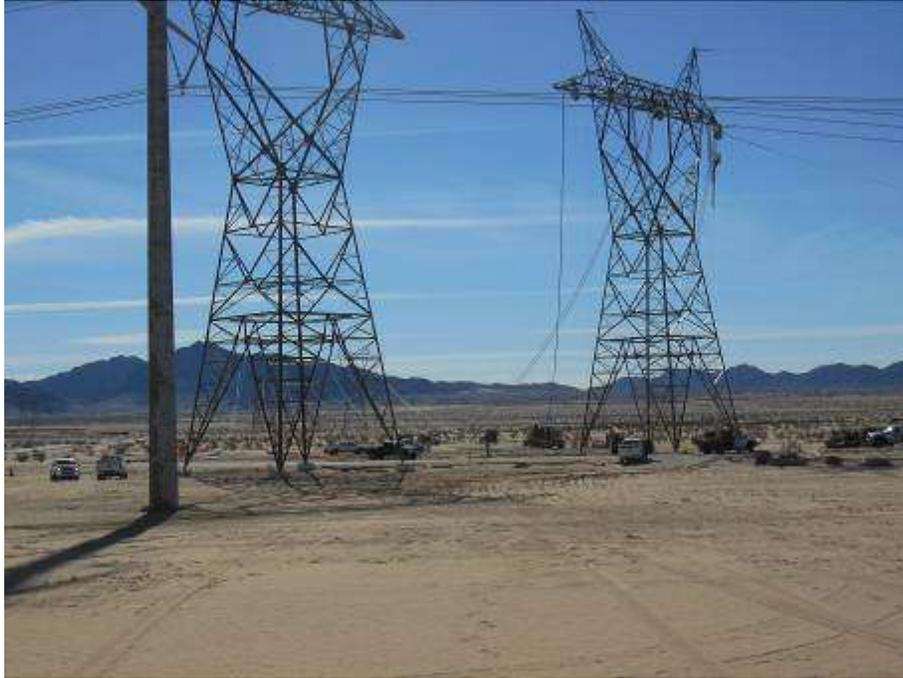
Figure 1. Wire stringing at Towers 2648 and CR1-1W.
