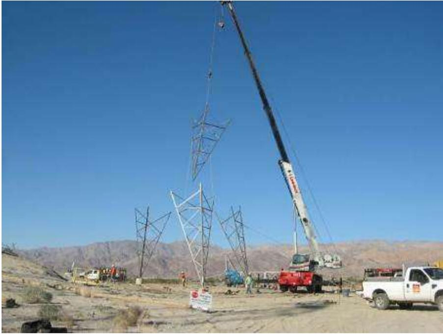
Figure 3. Steel erection at Tower 2246.
