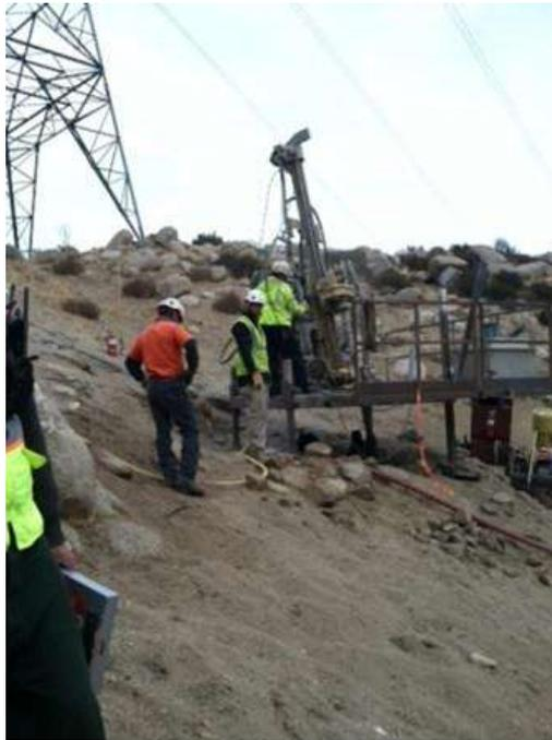
Figure 4. Micropile drilling at Tower 1038.
