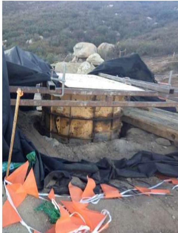
Figure 8. Improperly covered excavation hole at Tower 1093. The hole was covered properly the previous day but wind conditions tore the felt material, leaving a large gap.
