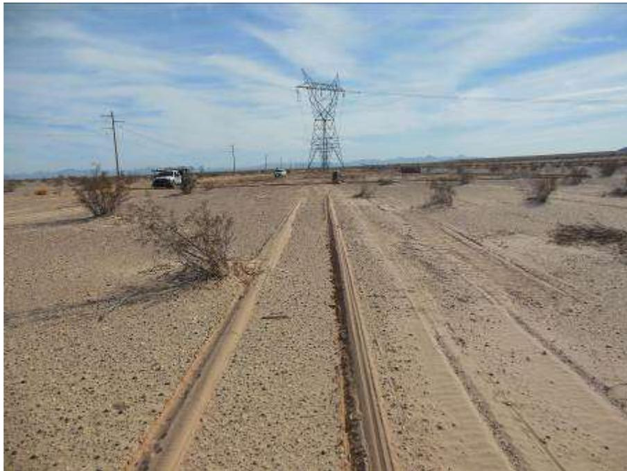
Figure 6. Ground disturbance associated with the removal of existing DPV1 conductor.
