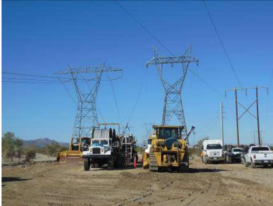
Figure 1. Set up of wire stringing equipment at Wire Site 77.
