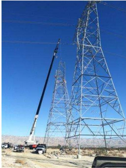
Figure 3. Tower assembly at Tower 2008.
