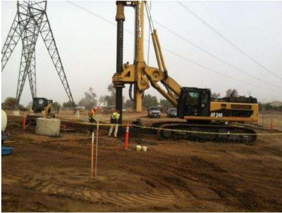
Figure 5. Foundation drilling at Tower 1147.
