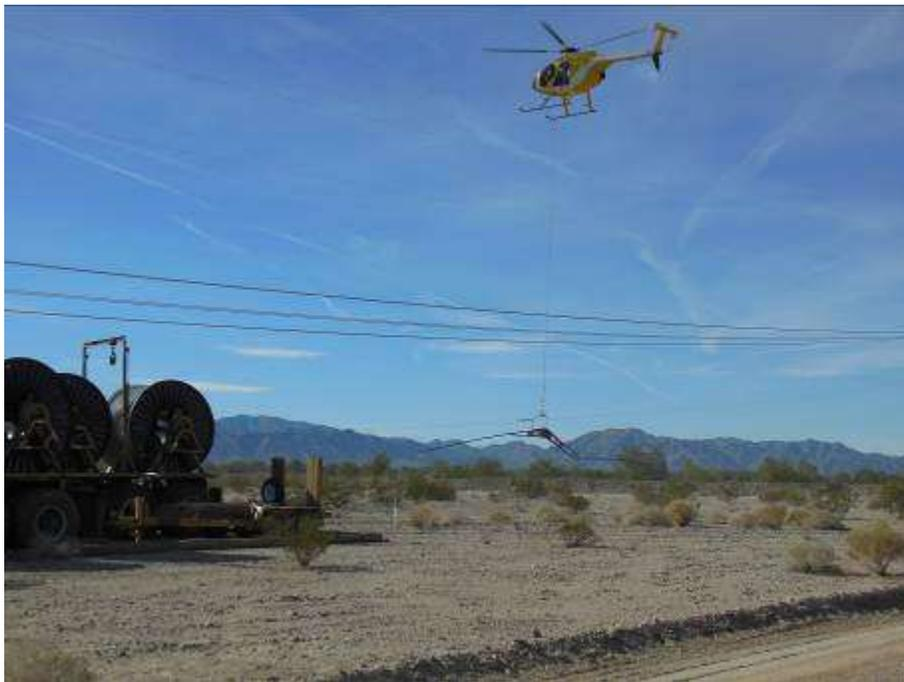
Figure 4. Wire stringing activities between the Red Bluff loop-ins and Tower 2539.
