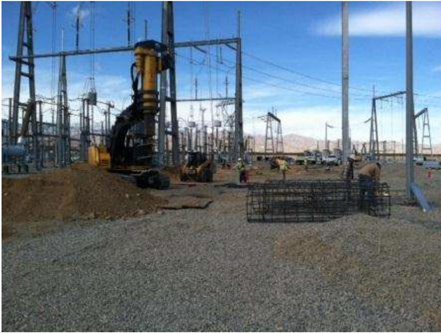
Figure 9. Foundation excavation for the 500 kV Switchrack within the Devers Substation.
