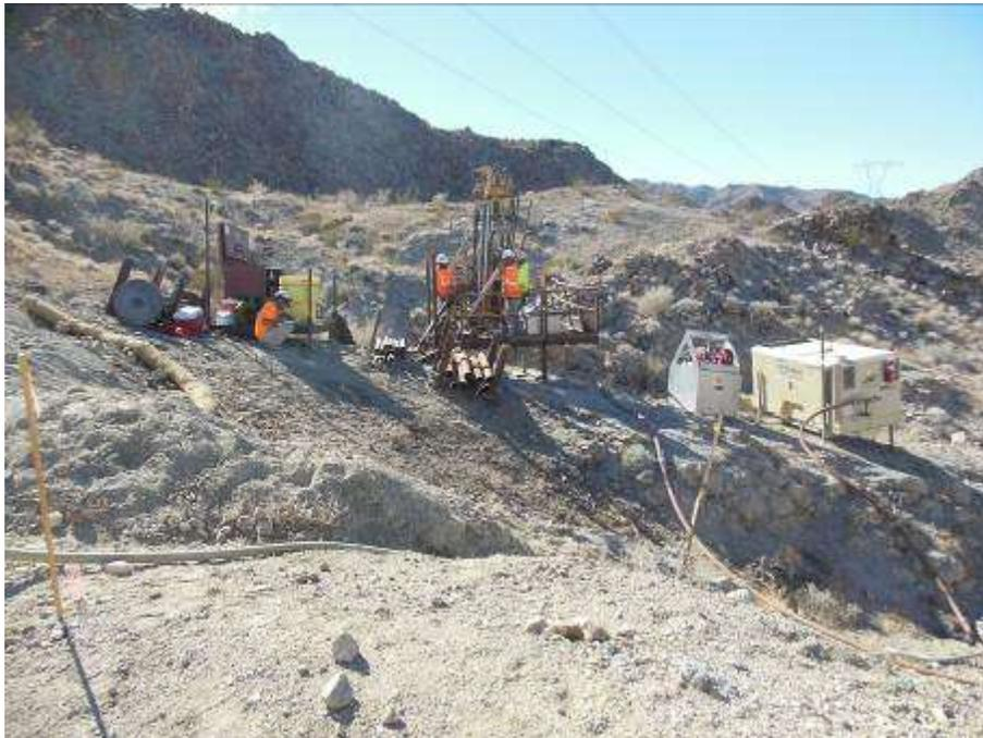
Figure 2. Micropile drilling at 2421.
