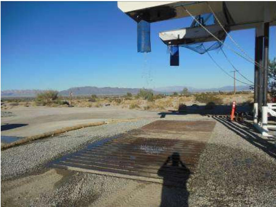
Figure 8. Water leaking from stand tank at Rice Road resulting in offsite sedimentation (note water flow outside of BMPs on left of photo).
