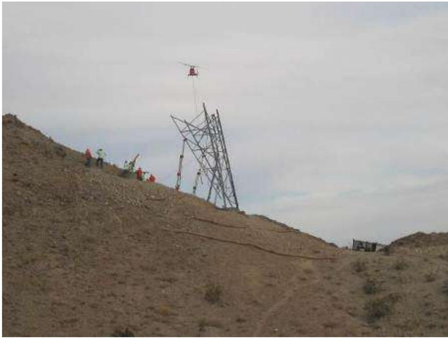
Figure 3. Micropile steel erection at Tower 2308.
