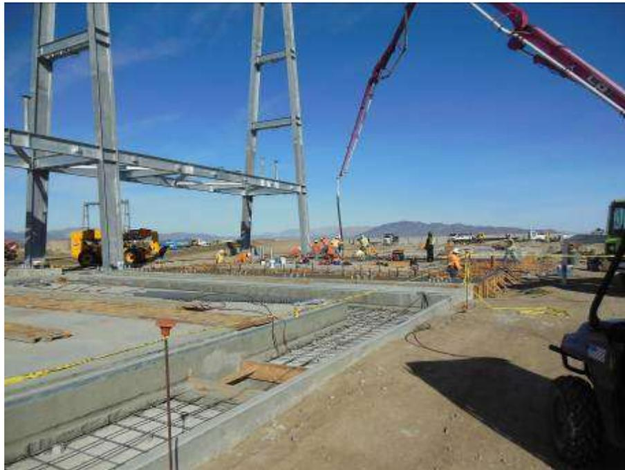
Figure 10. Transformer pad and switchrack construction at Red Bluff Substation.
