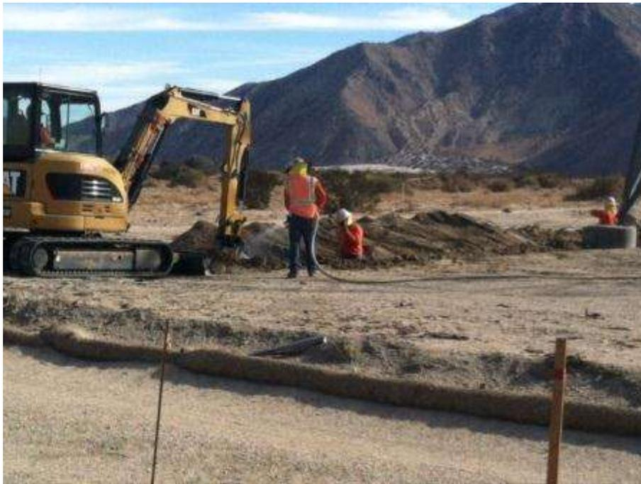
Figure 6. Ground wire trenching at Tower 1024.
