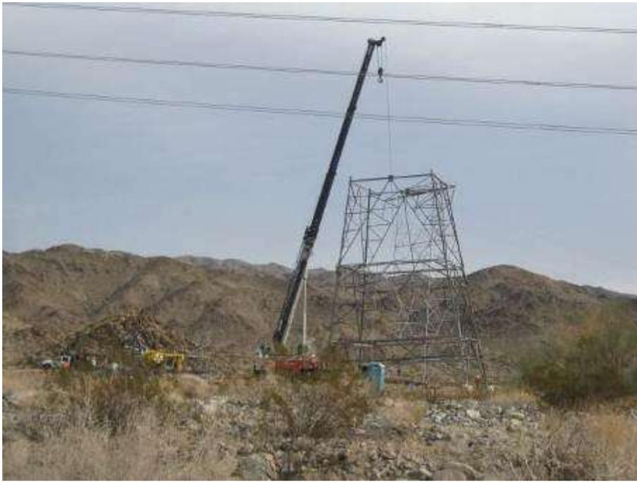
Figure 3. Steel erection at Tower 2326ALT.
