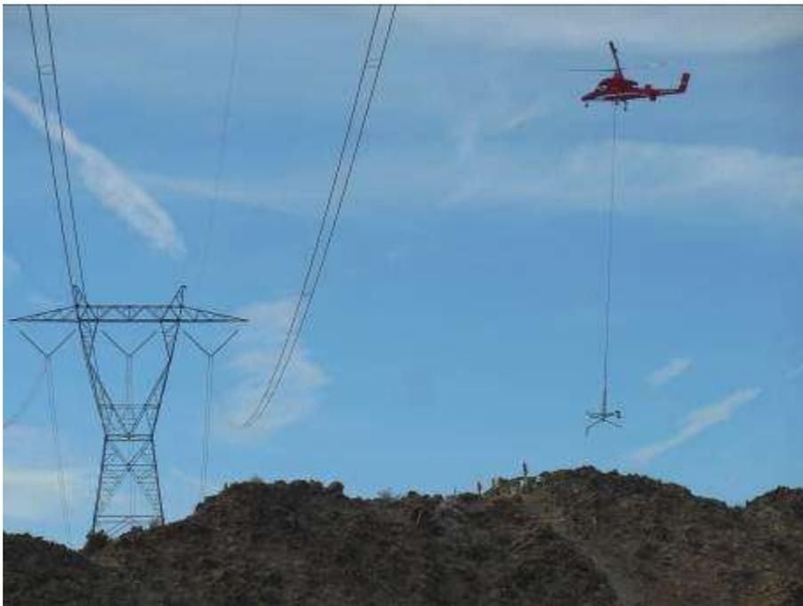
Figure 4. Transfer of assembly material from HLZ H5 to Tower 2424.
