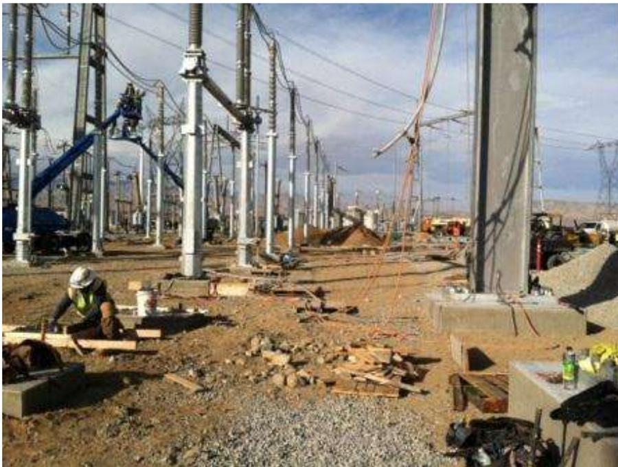
Figure 8. Foundation work and installation of switchracks within the expansion area of Devers Substation.
