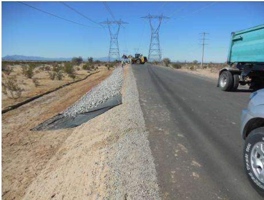
Figure 10. Installation of riprap along CRS access road.
