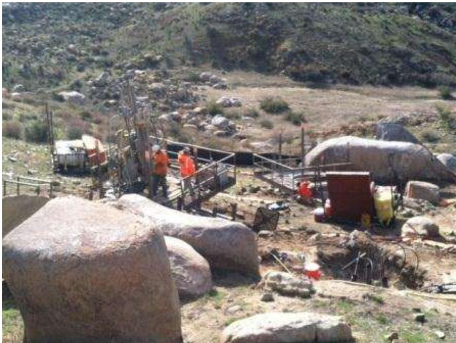
Figure 6. Micropile drilling at Tower 1074.
