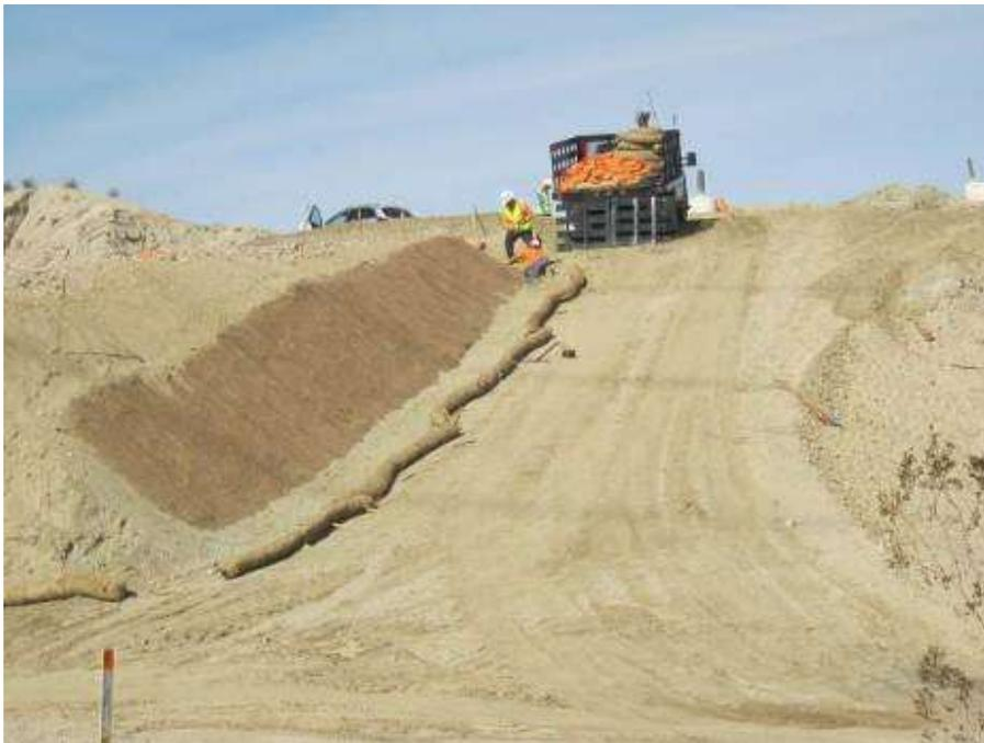
Figure 2. BMP jute netting installation on side slope at Tower 2234.
