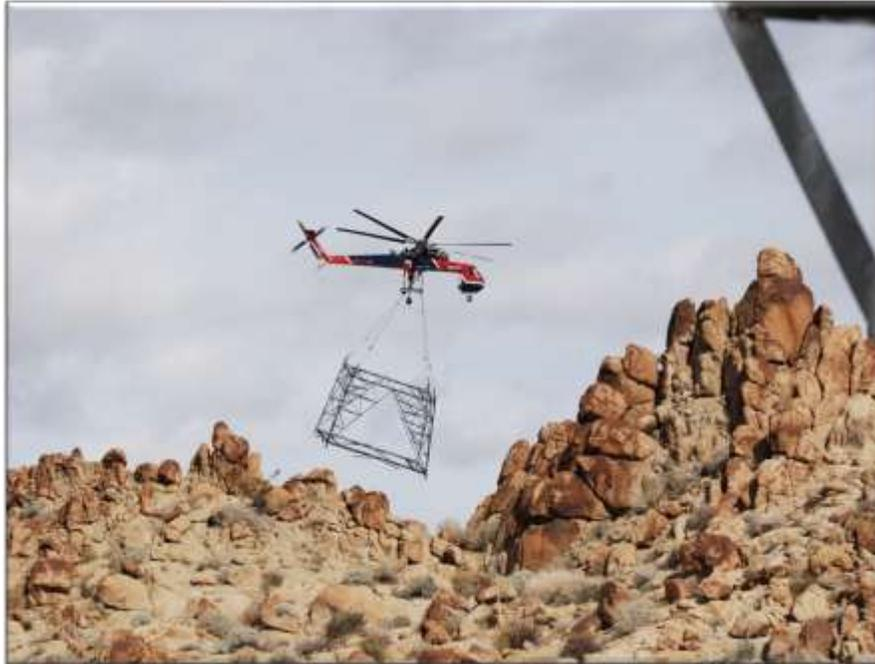
Figure 4. Transporting tower laybacks to Tower 2425 via Skycrane.
