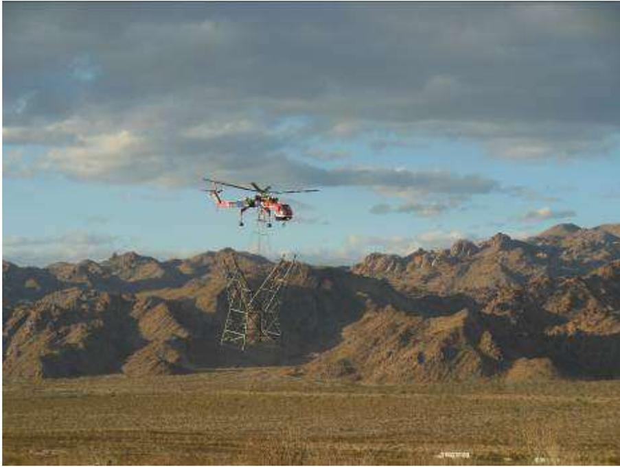
Figure 3. Transporting tower laybacks between HLZ H4 and Tower 2412 via Skycrane.
