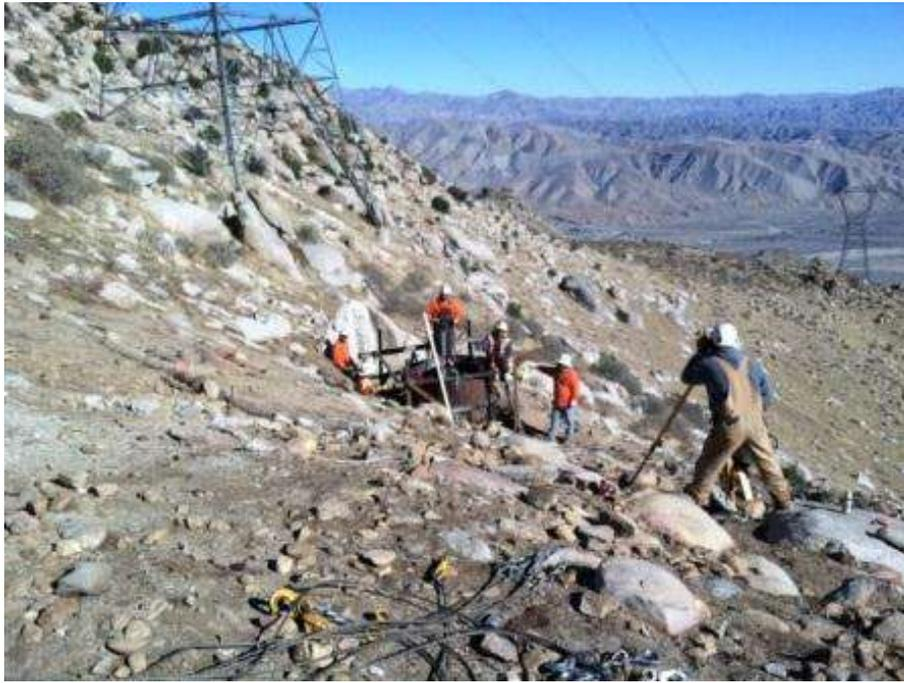
Figure 7. Pilecap set-up for micropile foundation at Tower 1039.
