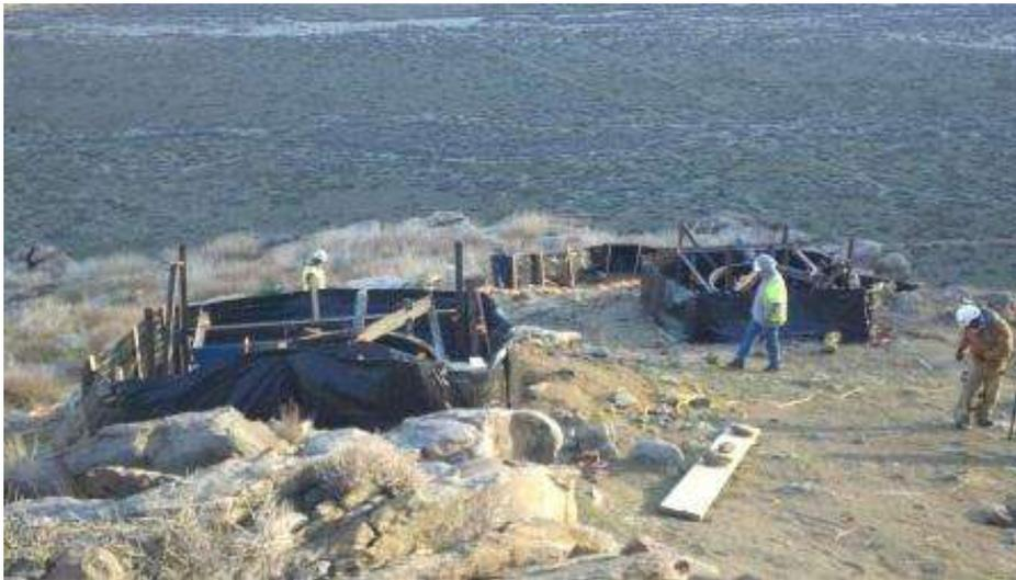
Figure 9. Silt fencing installed around micropile foundation excavations at Tower 1067 to prevent wildlife entrapment.
