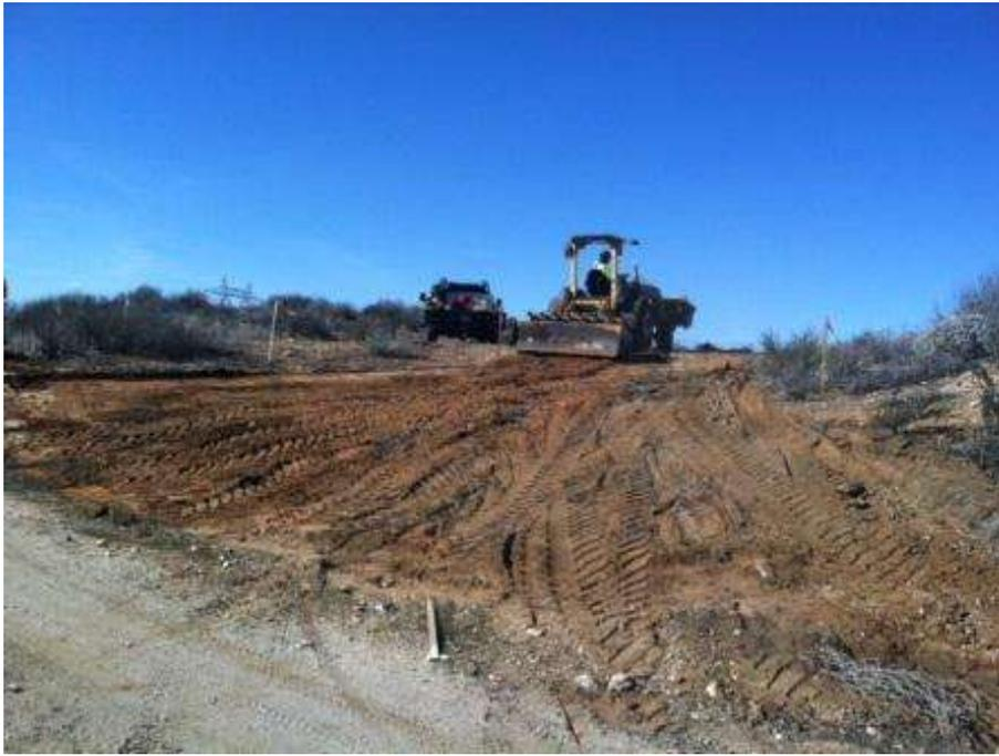
Figure 3. Site clearing and grading at Tower 1131.
