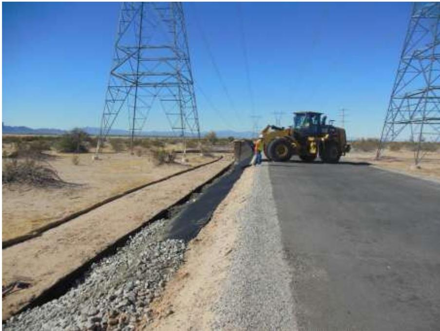
Figure 6. Key trenching and installation of riprap along CRS access road.
