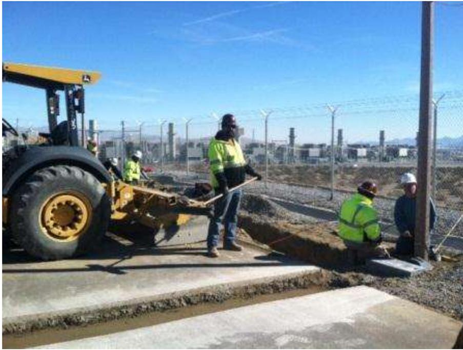
Figure 9. Trenching work for lighting installation within the Devers Substation expansion area.
