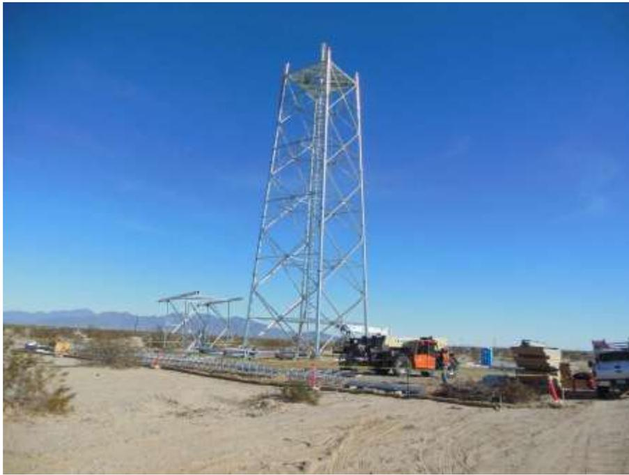
Figure 7. Erection of the telecomm tower at the Desert Center site.
