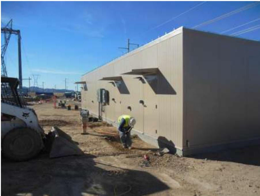
Figure 8. Installation of the MEER building at the Series Capacitor site.
