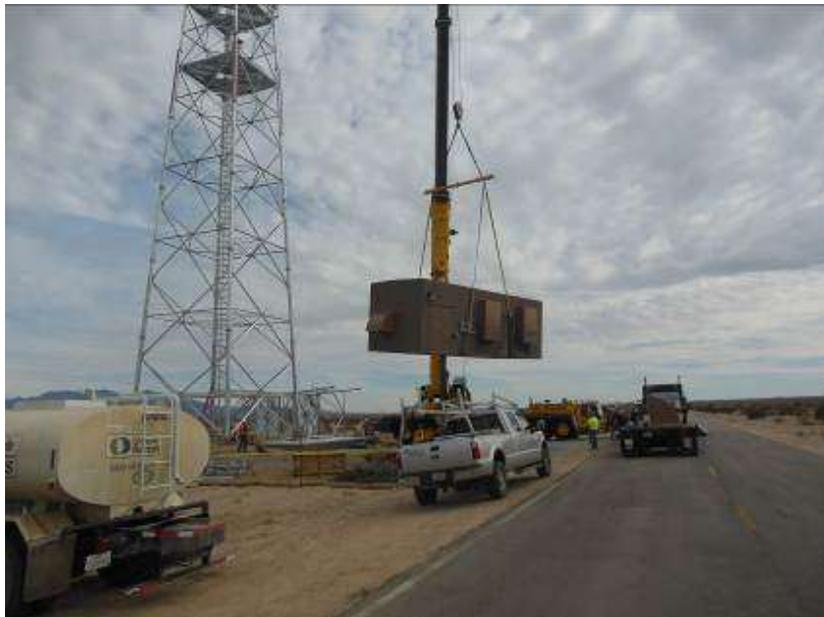
Figure 10. Installation of the MEER building at the Desert Center telecomm site.
