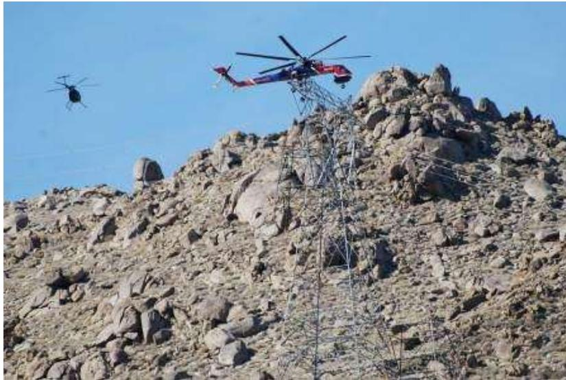
Figure 5. Tower assembly using a skycrane between Towers 1032-1036 (photo courtesy of SCE).
