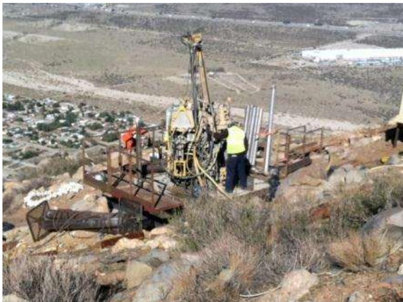
Figure 4. Micropile drilling activities at Tower 1050.
