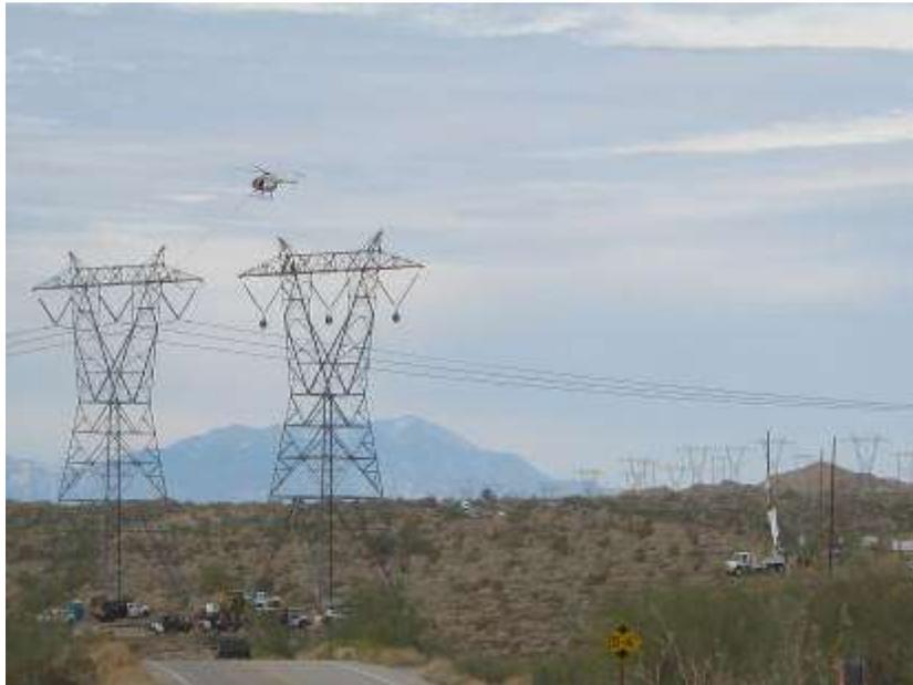
Figure 2. Pulling sockline at Tower 2327.
