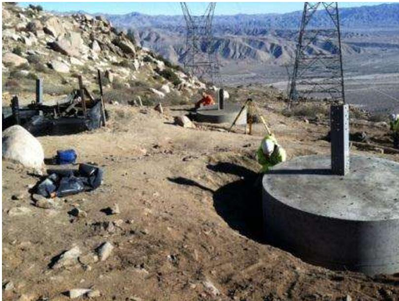
Figure 6. Micropile foundation finishing at Tower 1040.
