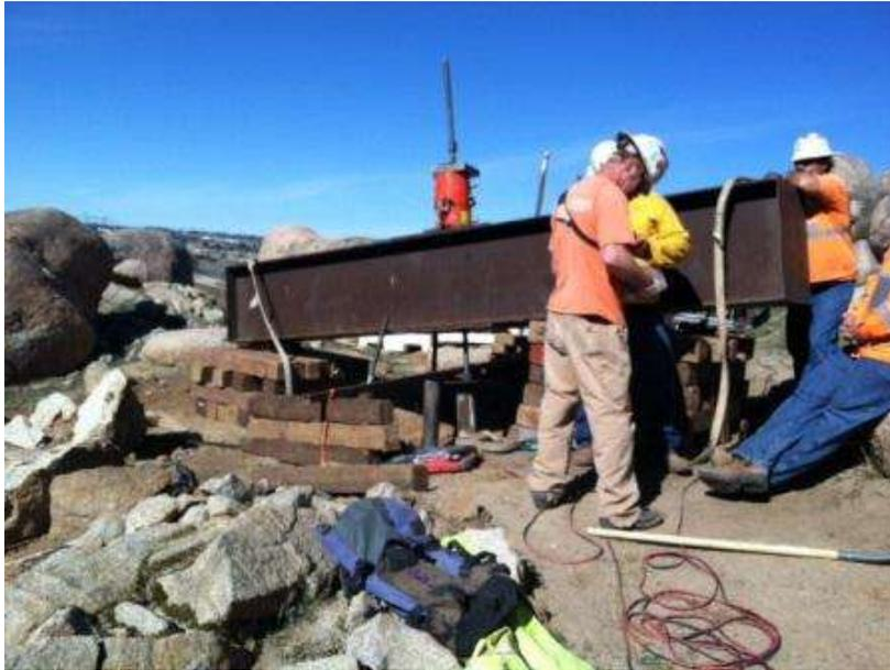
Figure 5. Micropile testing at Tower 1074.
