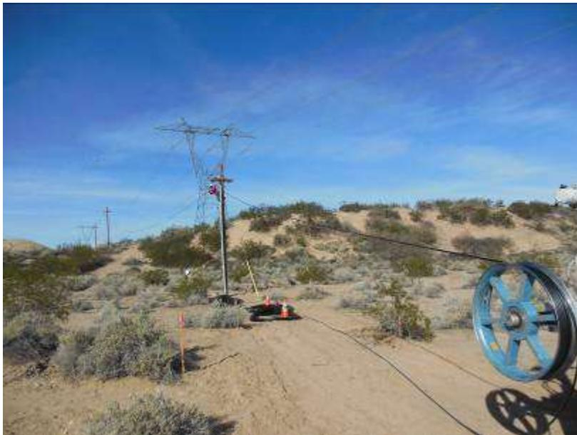
Figure 8. Pulling above ground wire along the Southeast Telecomm Line.
