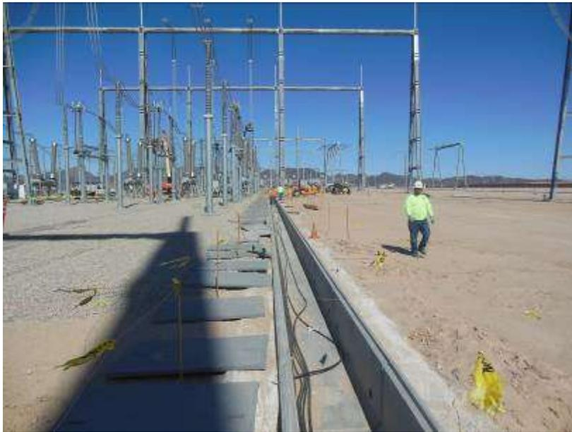
Figure 7. Installation of conduit at CRS.
