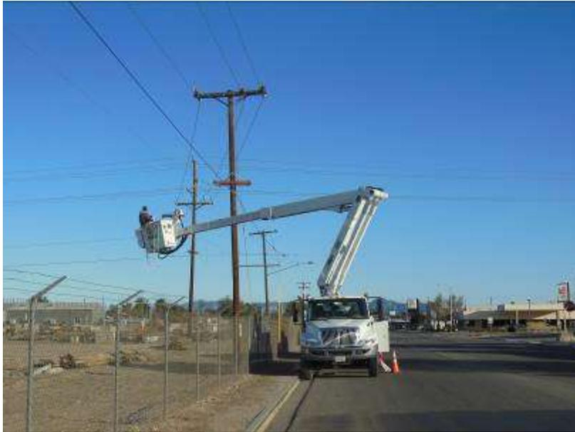
Figure 9. Wire stringing from bucket truck along SE Telecomm line.
