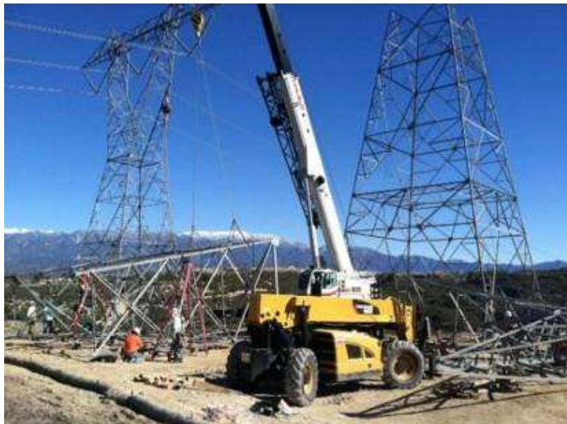
Figure 4. Steel assembly at Tower 1098.
