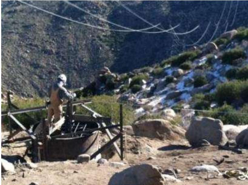
Figure 5. Pilecap preparation at Tower 1044.
