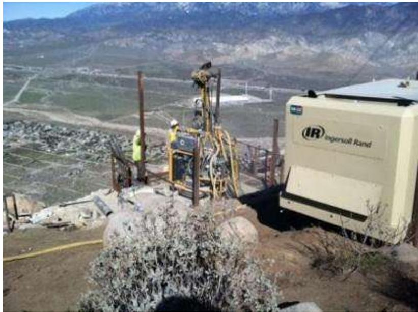
Figure 3. Micropile drilling at Tower 1049.
