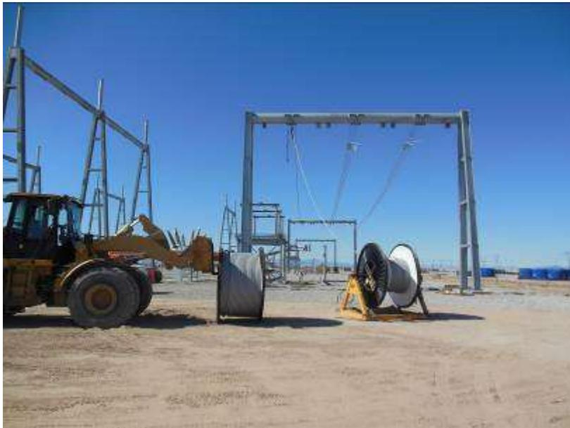
Figure 8. Stringing wire along switchrack at CRS.
