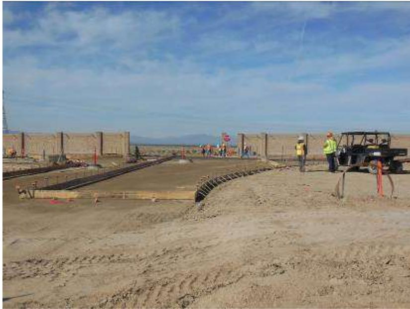
Figure 7. Foundation work associated with the driveway at CRS.
