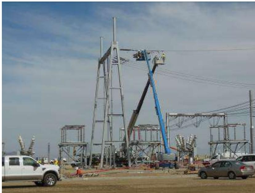
Figure 8. Wire stringing at Red Bluff Substation.
