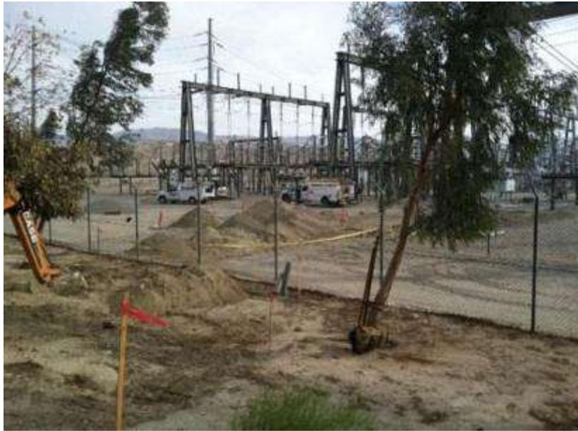
Figure 9. Trenching activities for the Mirage Loop-ins inside and outside of the Mirage Substation.
