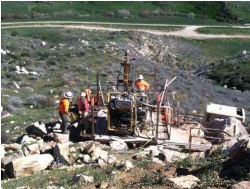
Figure 4. Micropile drilling activities at Tower 1112.
