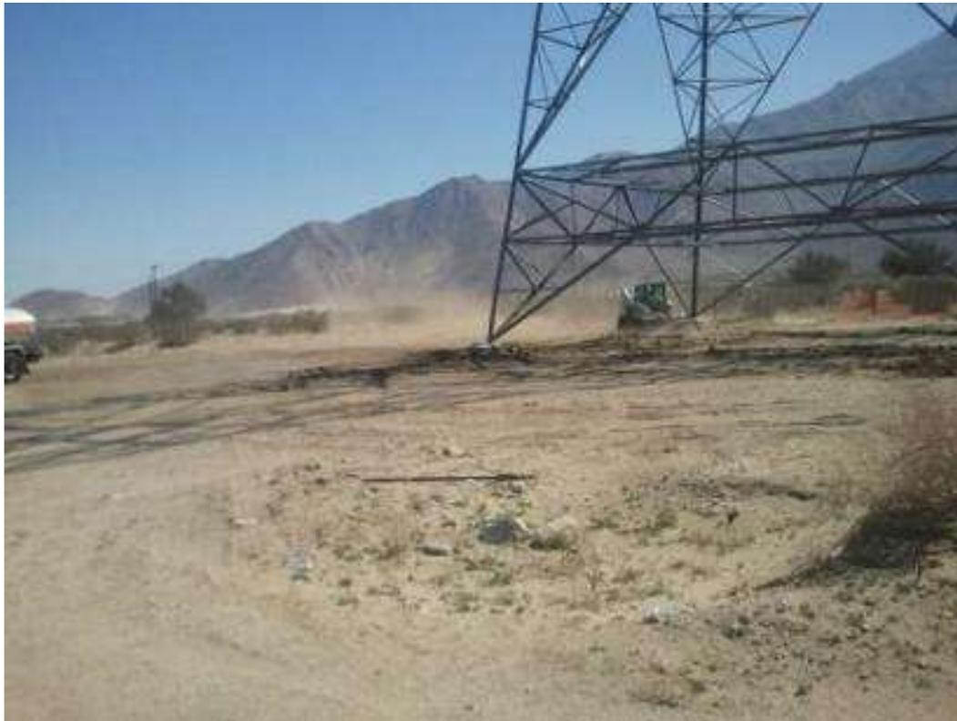
Figure 4. Fugitive dust observed at Tower 1025 during foundation close-out activities. Photo courtesy of FRED.
