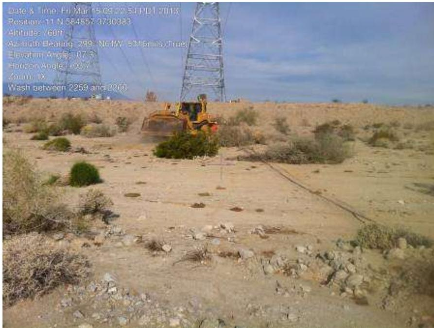
Figure 7. After the conductor fell to the ground, it was decided to mobilize one bulldozer on an existing off-road trail (selected by the SCE Biologists to minimize impacts) located in a large wash immediately west of the wire/pull site. Crews were able to temporarily secure the wire. (Photo courtesy of FRED).
