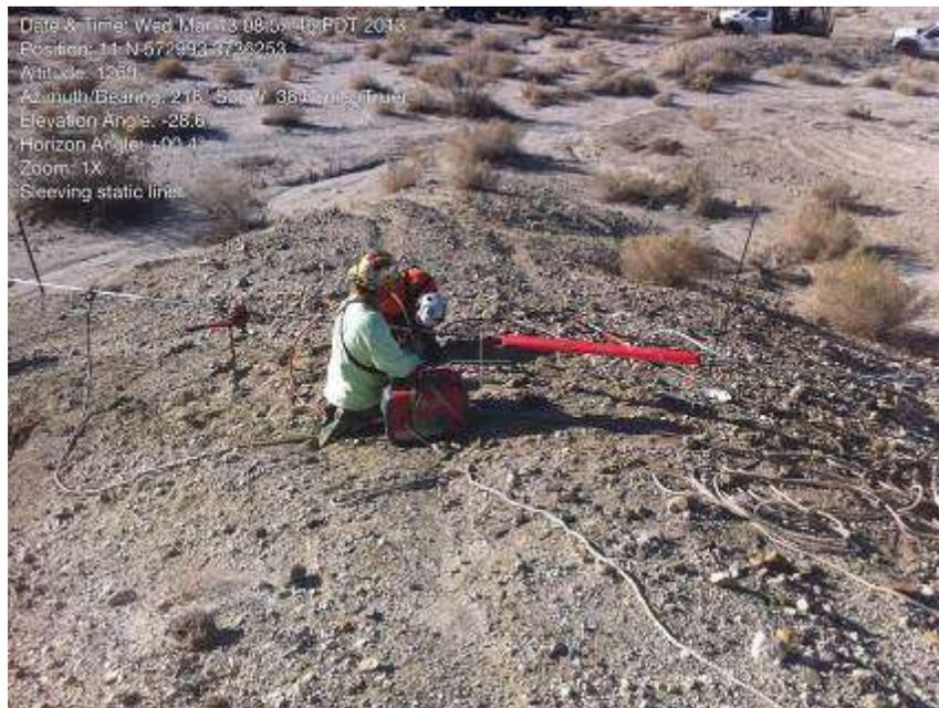
Figure 4. OPGW crew conducted sleeving of the static wire outside the approved disturbance areas between Towers 2230 and 2230AX. (Photo courtesy of FRED)
