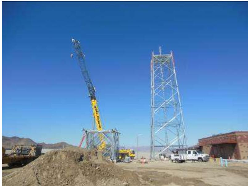
Figure 6. Steel erection of the telecomm tower at Red Bluff Substation.
