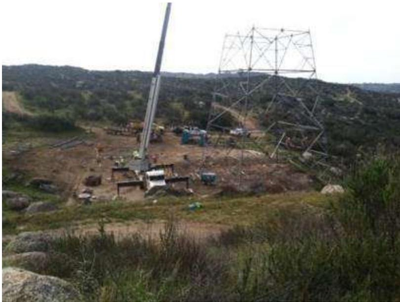
Figure 3. Tower assembly at Tower 1130.
