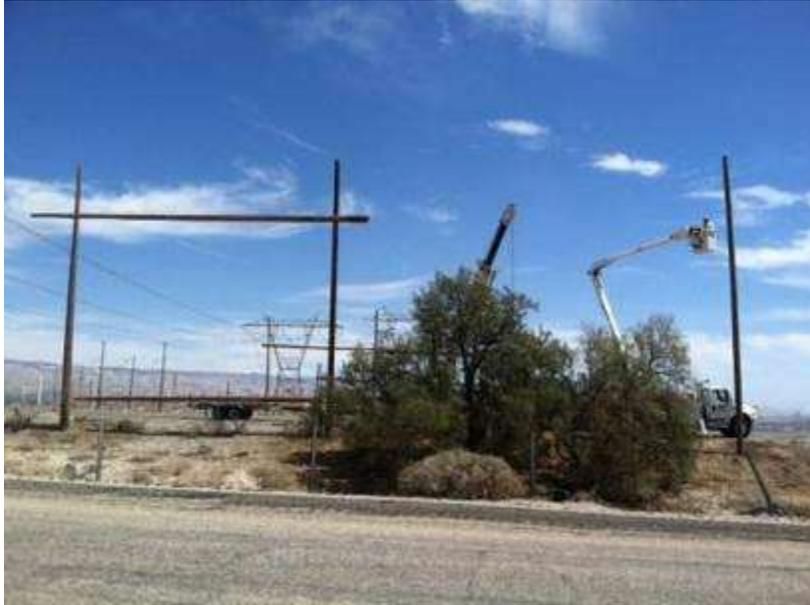
Figure 1. Installation of Guard Poles at GS12 next to HWY 62.
