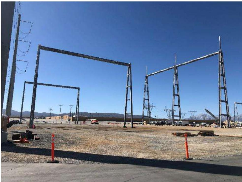
**Photo 2:** Dead-end structure A-Frames within Lugo Substation. View southeast. (February 25, 2021).
