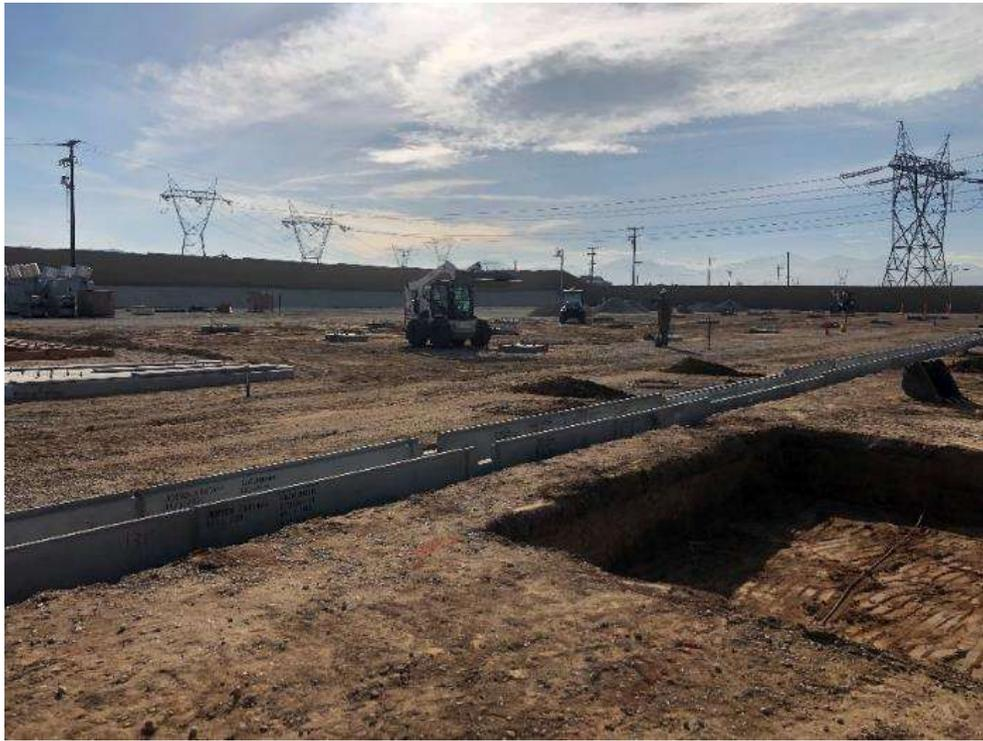
**Photo 1:** Burial of trenching for grounding wire at Lugo Substation. View southwest. (February 11, 2021).
