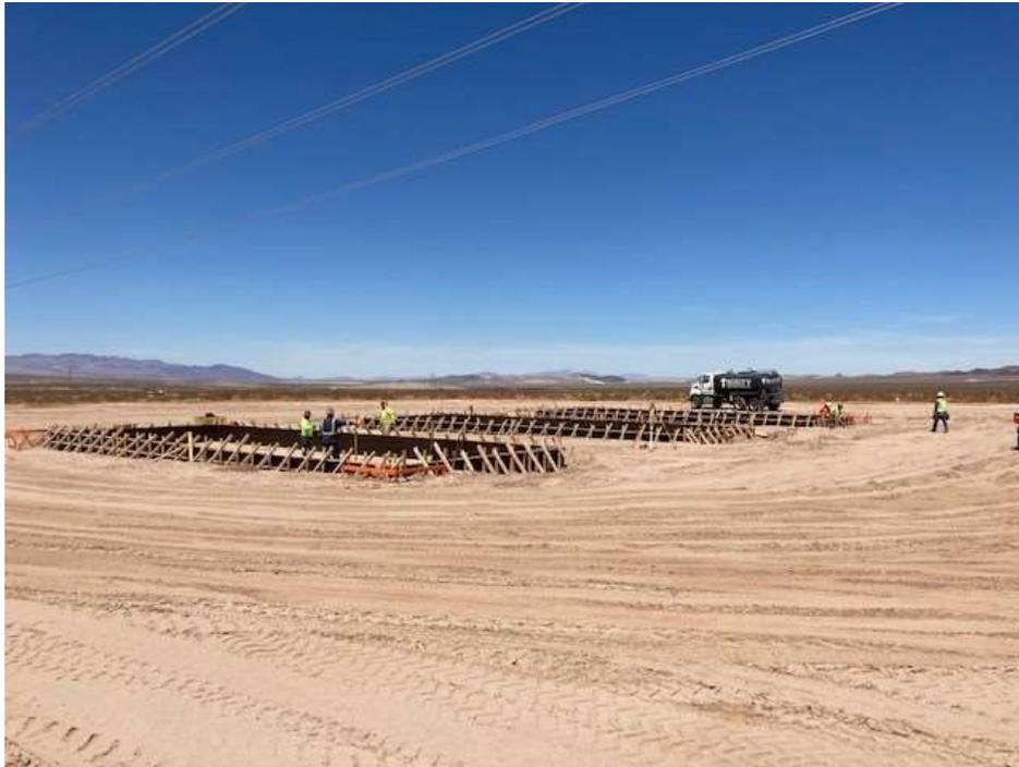
**Photo 3:** Forming concrete pads at the Ludlow Series Capacitor. April 29, 2021.
