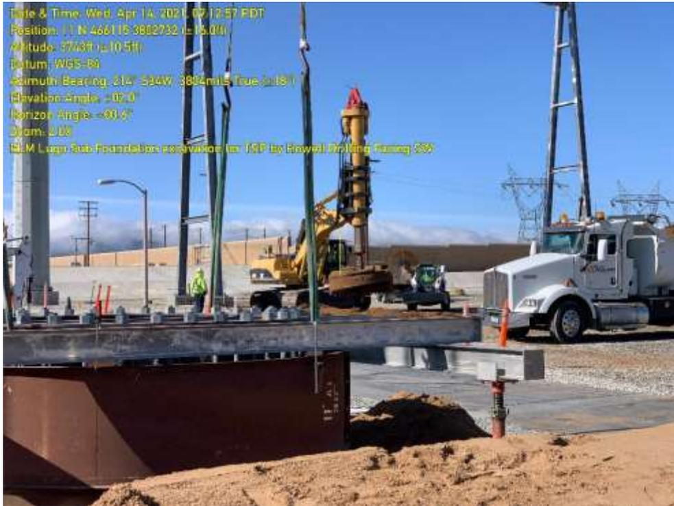
**Photo 1:** Drilling for foundations at the Lugo Substation. April 14, 2021. Photo courtesy of SCE.
