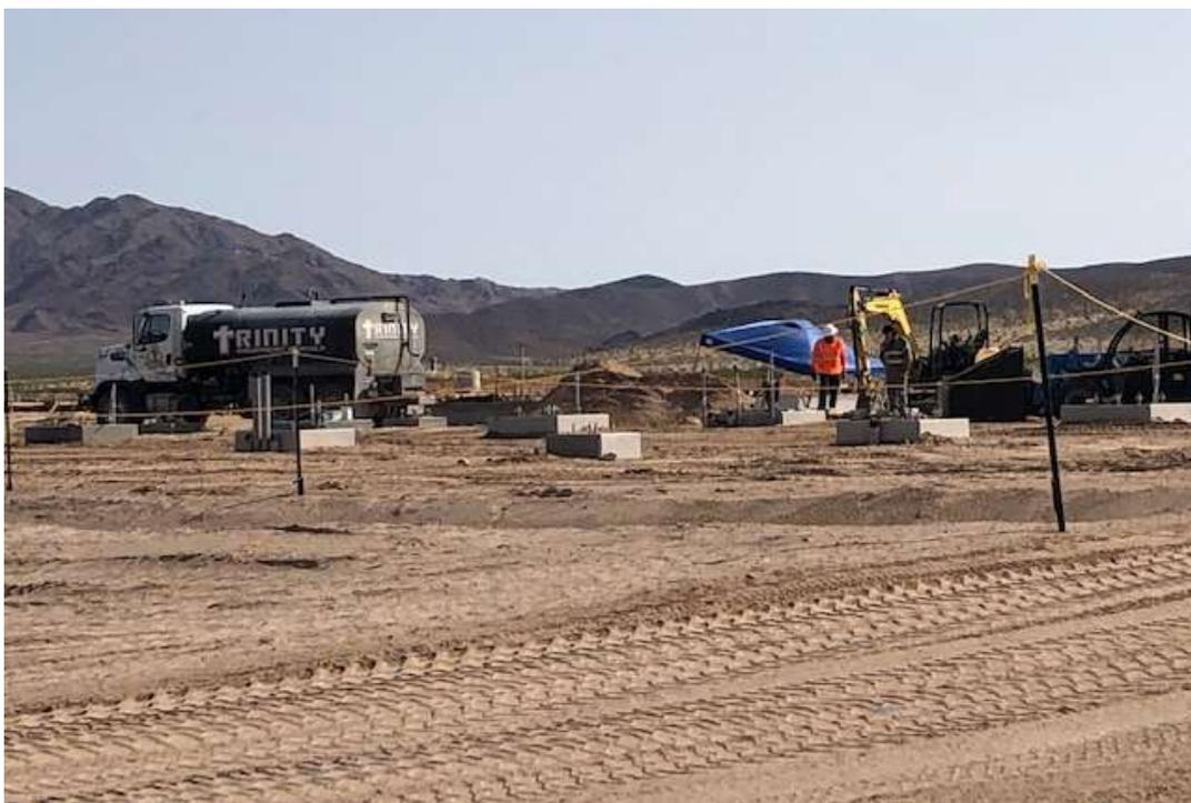
**Photo 2:** Excavating foundations at Ludlow Series Capacitor (August 12, 2021).
