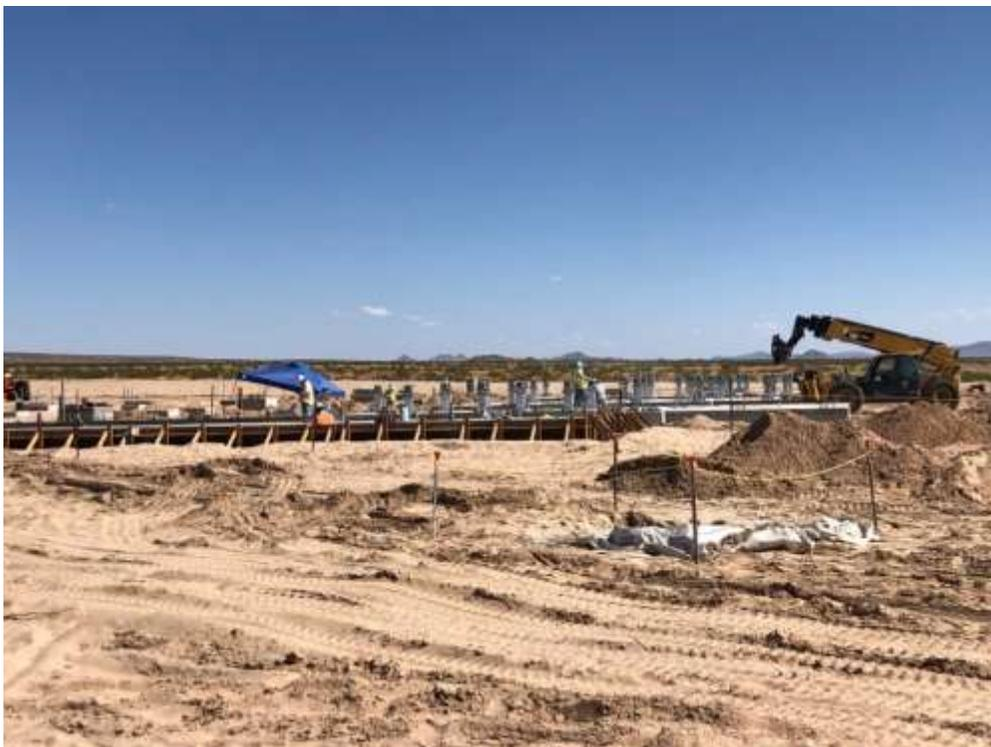
**Photo 2:** Excavating foundations at Ludlow Series Capacitor (September 2, 2021).
