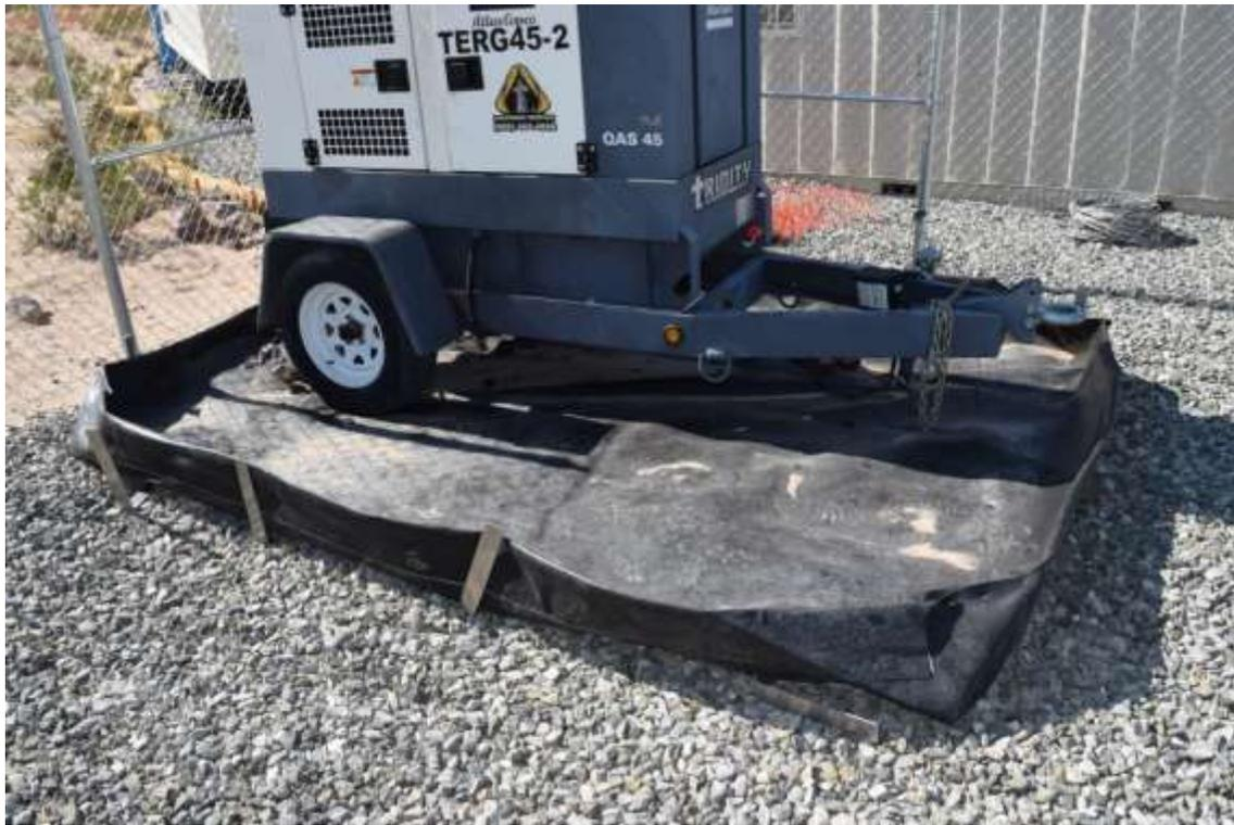
**Photo 5:** Repaired secondary containment and leaky generator at Ludlow Midline (September 14, 2021). Photo courtesy of SCE.
