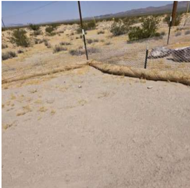
Photo 1: Slightly damaged perimeter wattles at SC2 (representative of conditions at SC5), with holes as a result of animal damage. Photo curtesy of the July 24, 2024 QSP SWPPP inspection.
