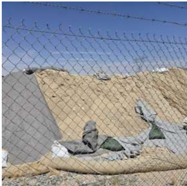
Photo 4: Damaged/large rip in stockpile covering (containing stockpiled soil) at SC2. The geo-tex fabric has torn apart across the top edge of this stockpile. Photo courtesy of the August 7, 2024 QSP SWPPP inspection.
