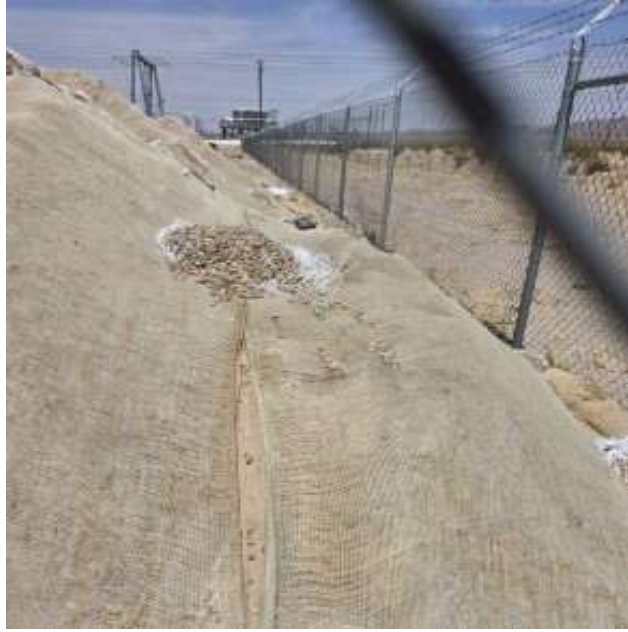
Photo 3: Damaged/large rip in stockpile covering (containing stockpiled soil) at SC2. Bags of gravel material put in place to secure the damaged covering also disintegrated. Photo courtesy of the August 7, 2024 QSP SWPPP inspection.
