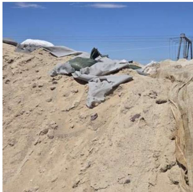
Photo 6: Damaged/large rip in stockpile covering (containing stockpiled soil) remains unaddressed at SC2. The geo-tex fabric has torn apart across the top edge of this stockpile. Photo courtesy of the August 21, 2024 QSP SWPPP inspection.
