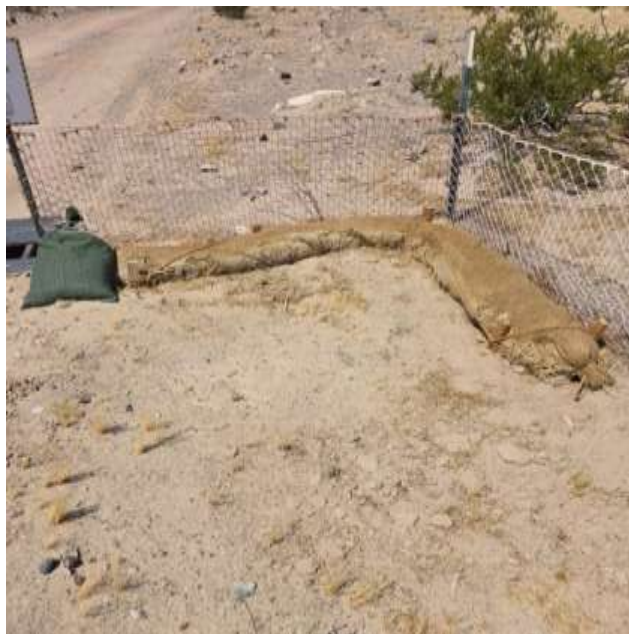
Photo 2: Damage to perimeter wattles, with a large split in the burlap covering at SC2. Photo curtesy of the July 24, 2024 QSP SWPPP inspection.
