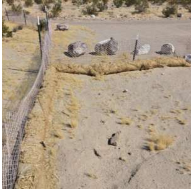
Photo 7: Significant damage to perimeter wattles at SC5, with loss of functionality as a BMP. Outstanding SWPPP maintenance needed/corrective action required. Photo courtesy of the September 25, 2024 QSP SWPPP inspection.
