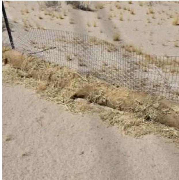
Photo 5: Significant damage to perimeter wattles at SC5, with a splits in the burlap covering, spill out of straw material, and loss of functionality as a BMP. Photo courtesy of the August 14, 2024 QSP SWPPP inspection.
