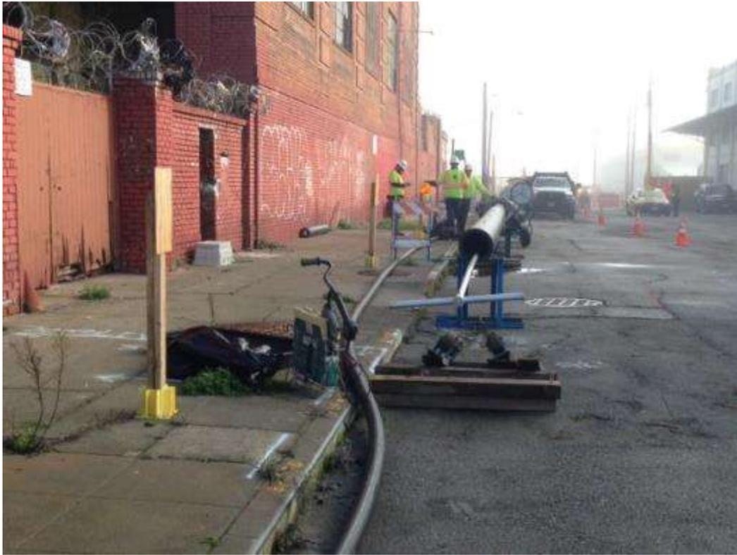
Figure 3 – HDPE fusing at HDD South along 23<sup>rd</sup> Street. View east, December 22, 2014.
