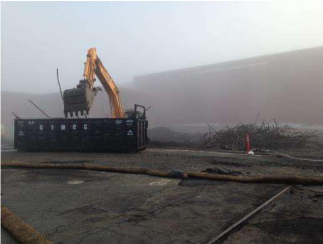
Figure 1 – Loading rebar to be hauled off and recycled at Potrero Switchyard. View northeast, December 22, 2014. Photo courtesy of PG&E.
