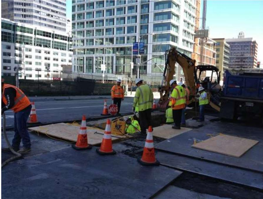
Figure 1 – Excavating duct bank trench on Folsom Street between 1<sup>st</sup> Street and Fremont Street. View northwest, September 8, 2015.
