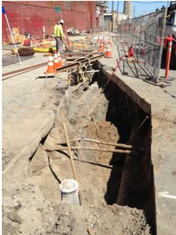
Figure 4 – Hand digging around utilities on 23<sup>rd</sup> Street. View east, September 8, 2015.
