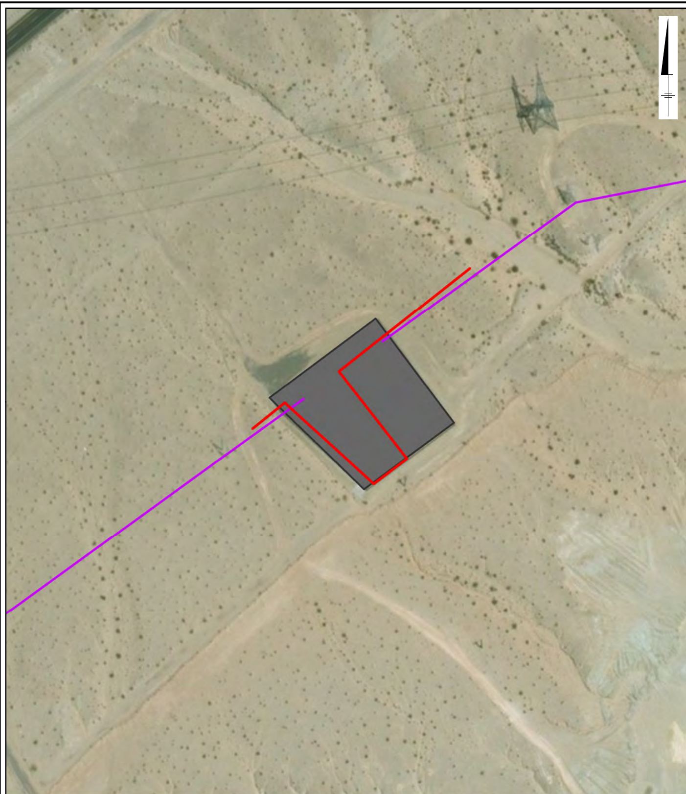
Dunn Siding Substation Page 9 of 12
