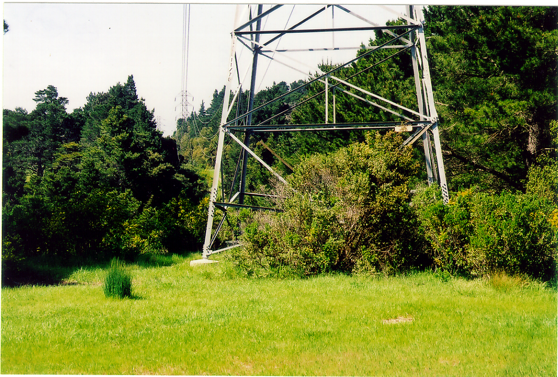
22. Woody vegetation under the towers is unsafe and needs to be removed.
