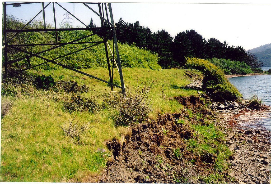
23. Shoreline erosion is occurring at Tower 13/83
