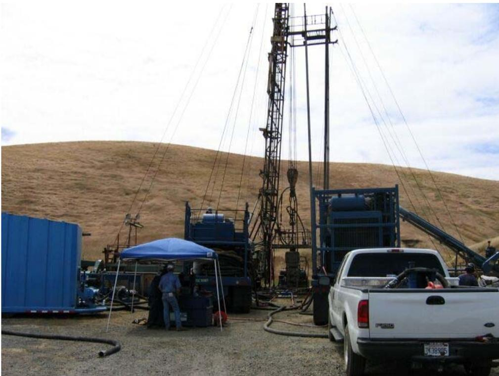
**Figure 2** – Work over rig at S-2 well site doing Frac and Pack work, June 13, 2006
