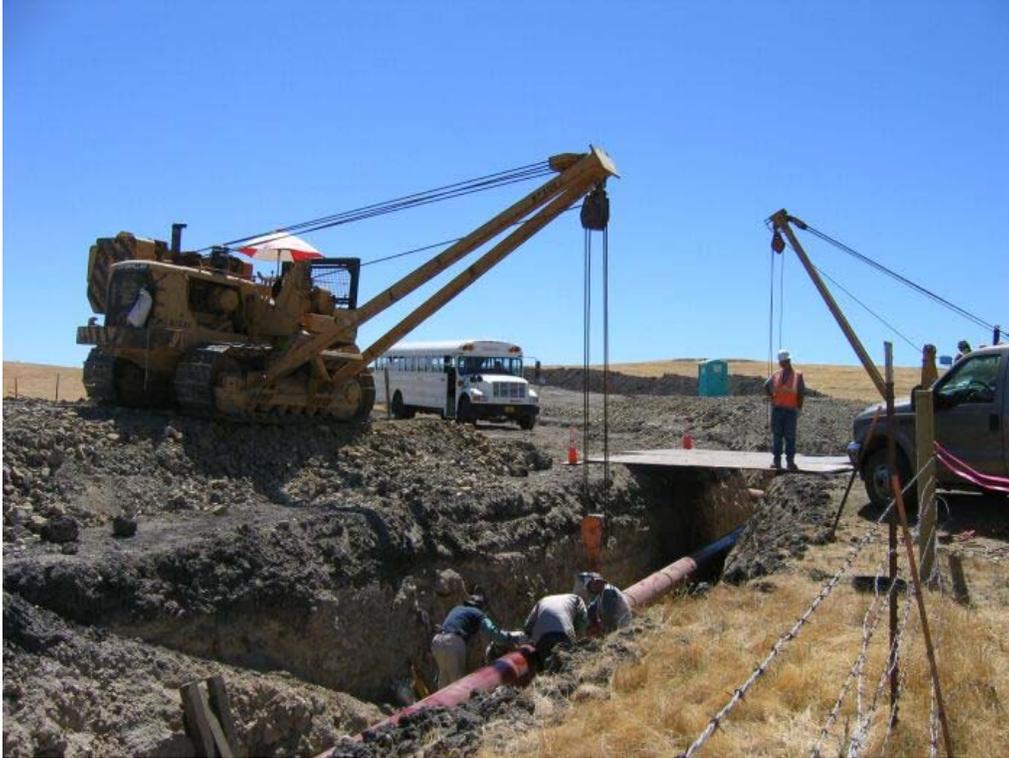
**Figure 1** – Crews welding 16-inch pipe near the “Y” in the access road to the Compressor Station, July 12, 2006.
