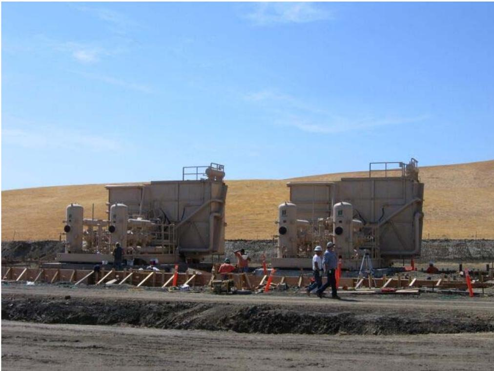
**Figure 3** – Foundation work around compressors at Compressor Station, September 21, 2006.
