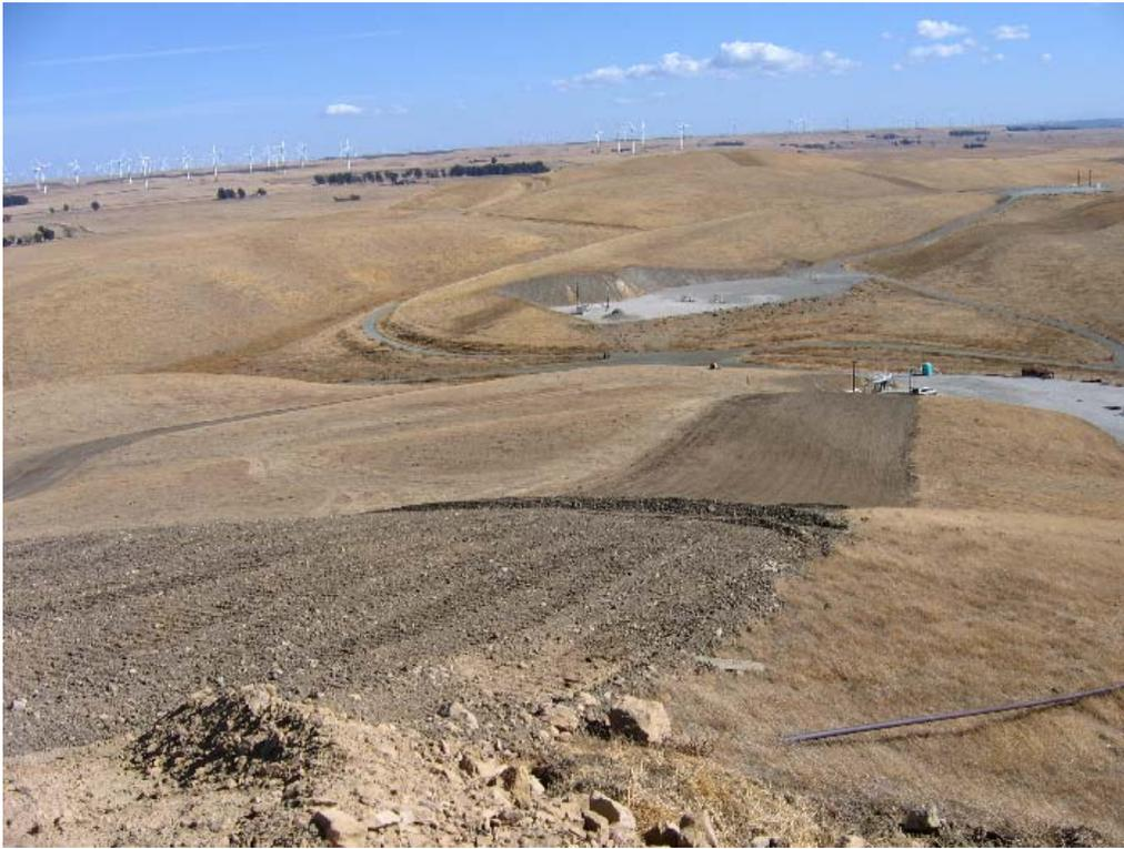
**Figure 3** – Backfilled pipeline right-of-way from Well Site S-5 down to Well Site S-2.
