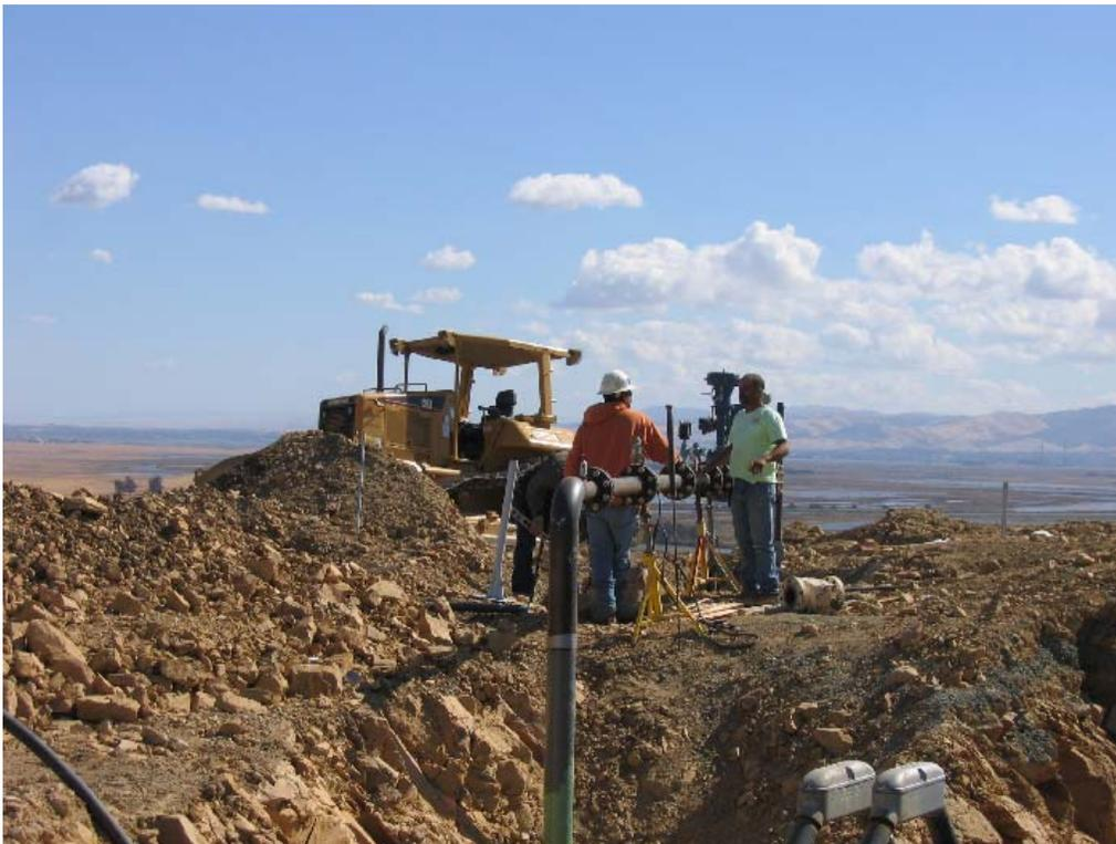
**Figure 2** – Crews conducting hydrostatic testing of pipe at Well Site S-5. October 4, 2007.
