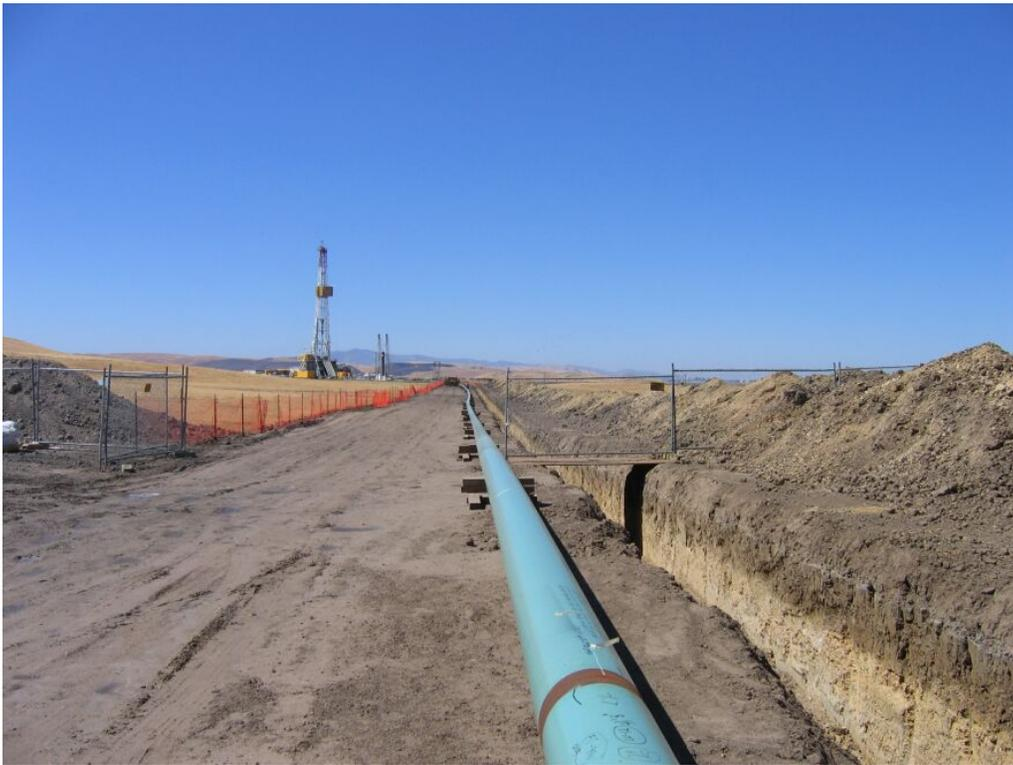
**Figure 4** – Pipeline pipe welded and set beside trench between the Compressor Station and WS-21, August 8, 2008.
