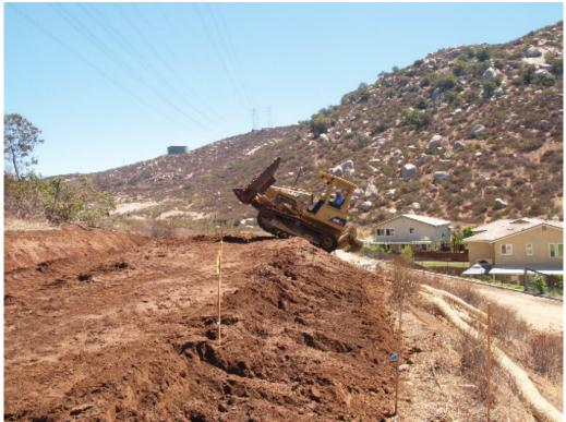
**Figure 3** – Small D4 bulldozer compacting side slope at Magnolia. Note the BMPs installed on the slope.
