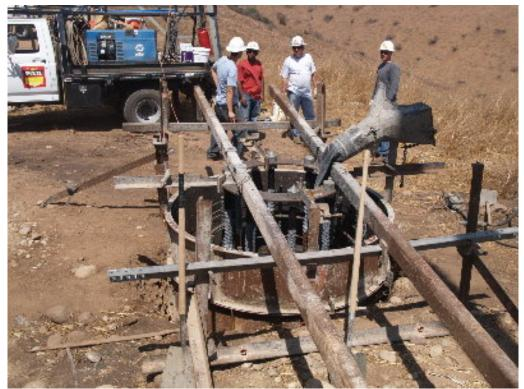
Figure 3 – Anchor bolts in place for concrete pour at Site 1400.
