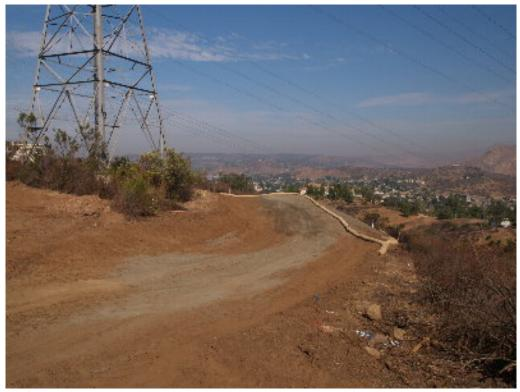
**Figure 6** – Pad completed with imported fill at Site 1101. Erosion control devices have been installed at the completed site.
