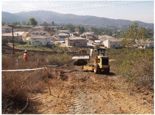
**Figure 5** – Operators placing and compacting imported fill at Site 1090 to bring pad up to engineered grade.
