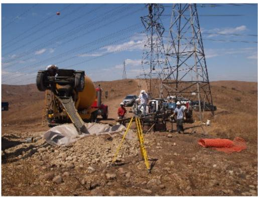
**Figure 4** – The PAR crew at Site 1400 constructed an effective concrete washout station for the concrete trucks.
