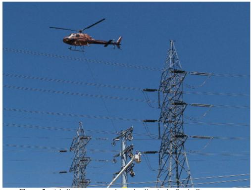
**Figure 5** – A helicopter was used to string line in the Steele Canyon area.
