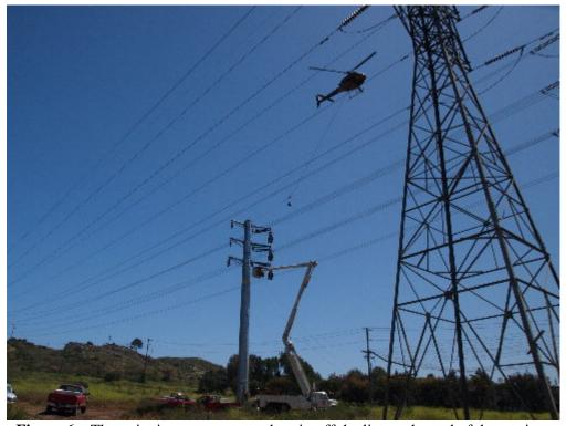
**Figure 6** – The stringing crew prepared to tie-off the line at the end of the section.
