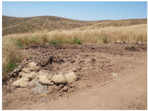
Figure 3 – The soil pushed off the access road at Fanita Junction needs to be cleaned and the area restored.
