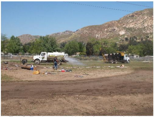
**Figure 7** – The string crew watered the right-of-way to control fugitive dust near residences.
