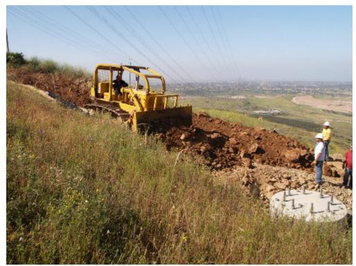
**Figure 1** – The PAR grading crew worked to prepare a pad for the crane on the access road.
