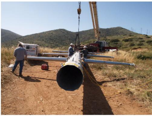
Figure 2 – The PAR crew worked on the access road to attach the arms to the upper section of a steel pole.
