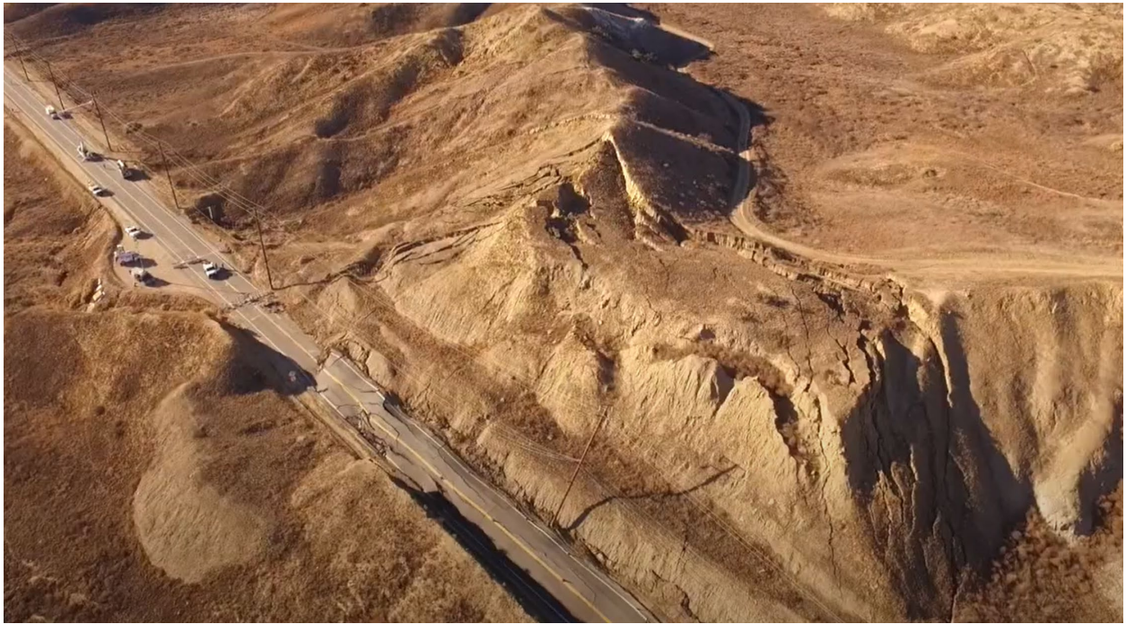
Vasquez Canyon Road Landslide Failure Plane and Roadway Uplift. November, 20, 2015. Source: https://youtu.be/Ef4e6eybLmk
