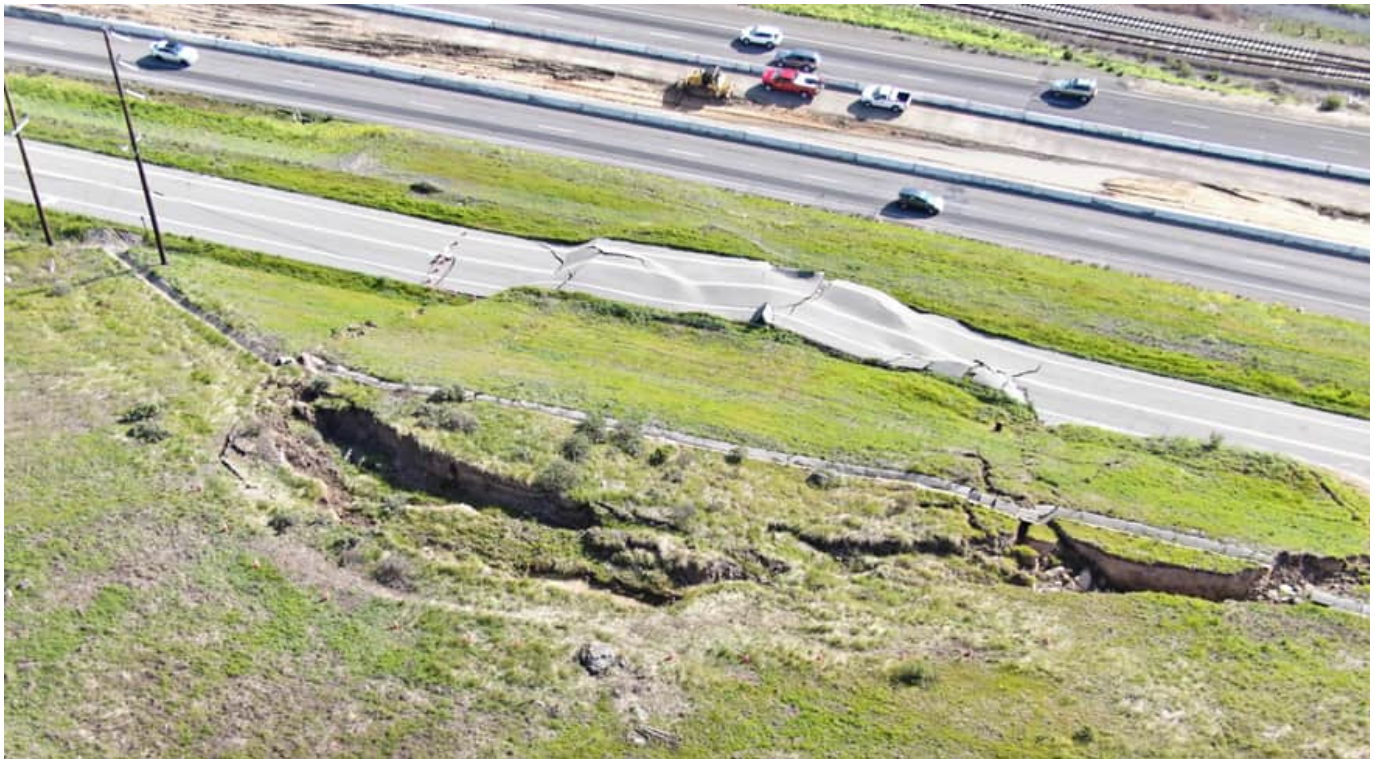
A deep-seated landslide with a failure plane extending under roadway.
