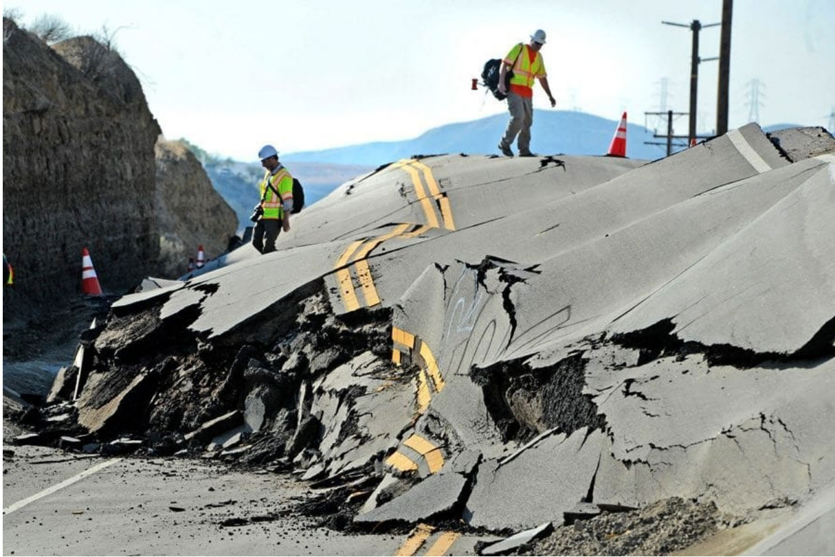
Los Angeles County Engineering Geologists climb on top of the buckled road where Vasquez Canyon Road has lifted up due to soil movement closing the road between Saugus and Canyon Country. Photo taken in November 2015 by Dan Watson, The Signal.
