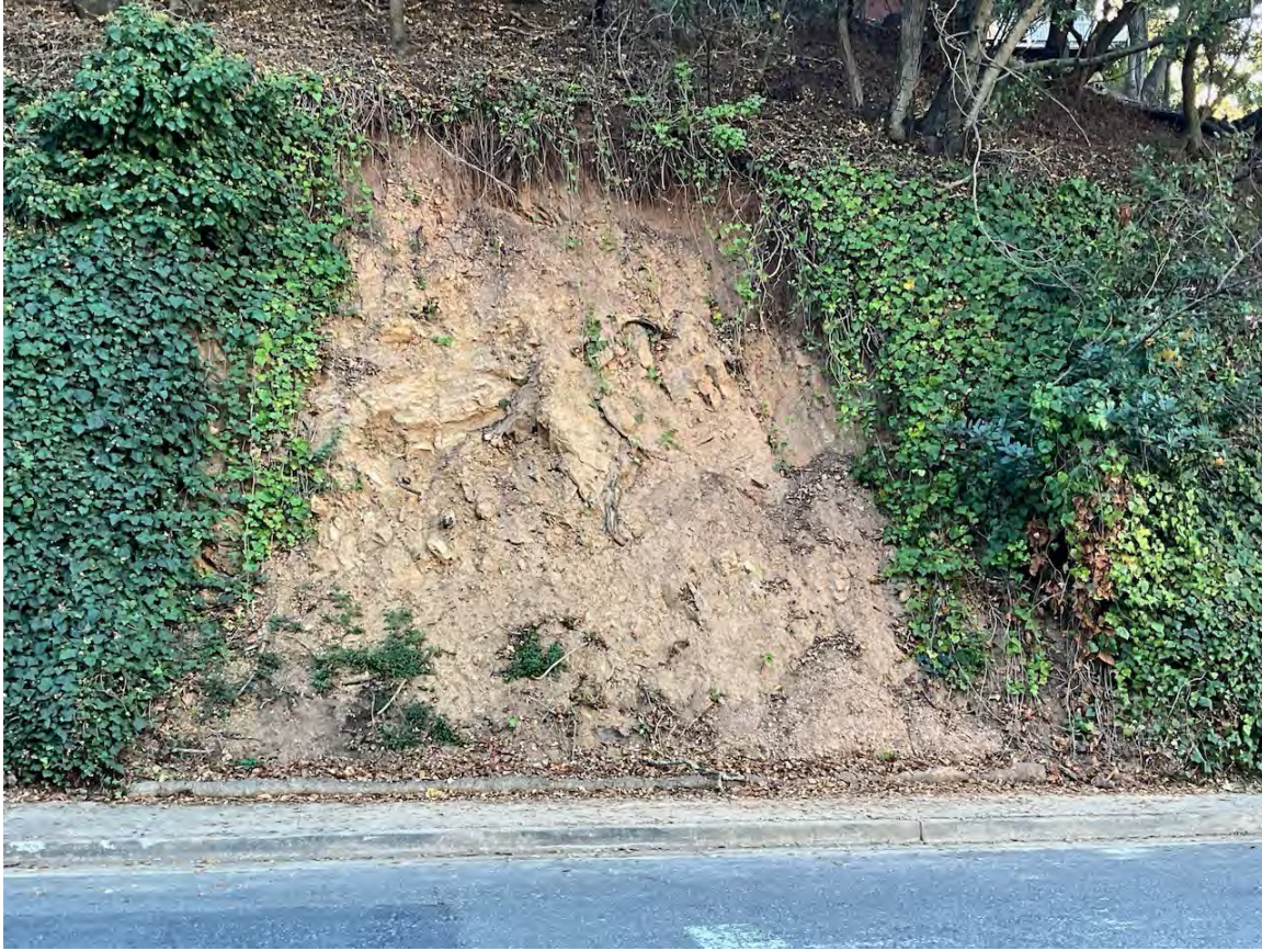
Photo 1: View southwest of recent shallow soil slip along overhead corridor on south side of Trestle Glen Road (See Figure 10 for location).
