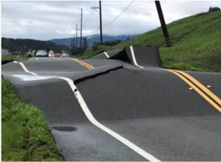
View of the approximate 3 to 4 feet of vertical displacement.
