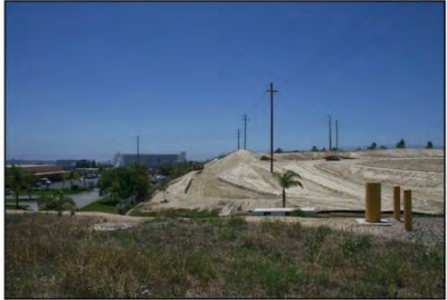
Northwest corner of Project Site, looking Northwest
