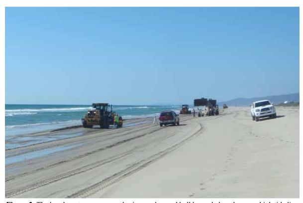
**Figure 2:** The beach route was prepared using graders and bulldozers below the mean high tide line to create an even driving surface for the crawler.
