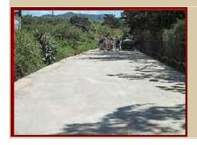
Crushed coral rock provides an attractive additional surface for a PX-300 road in Japan.
