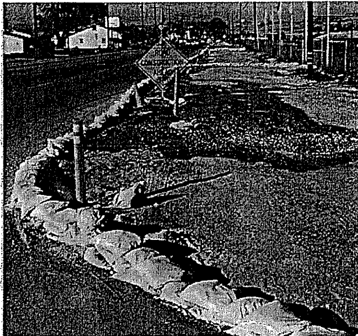
Sand bags used as perimeter control.
