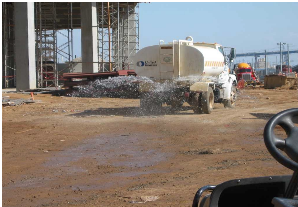
Water being applied for dust control.
