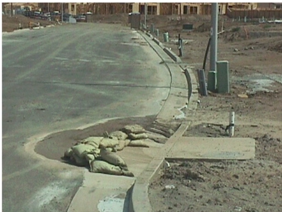
Gravel bag inlet protection.
