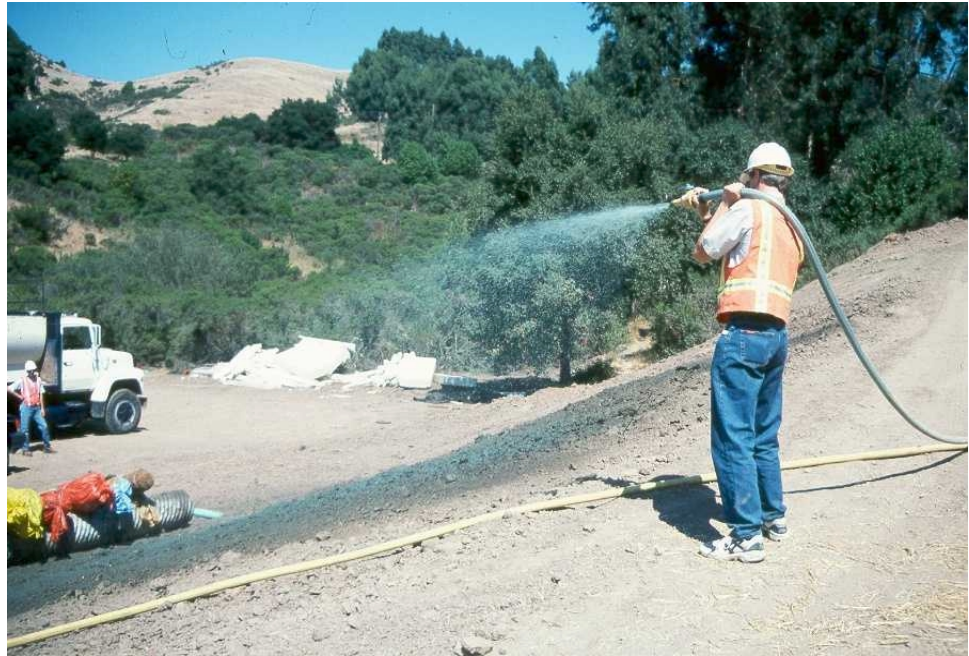
Applying hydroseed.
