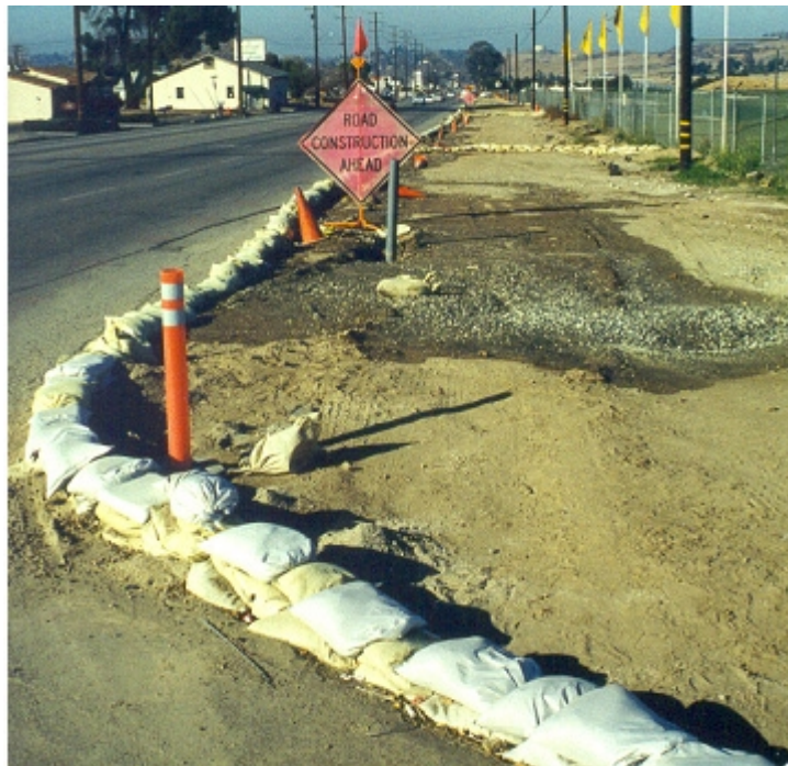
Sand bags used as perimeter control.
