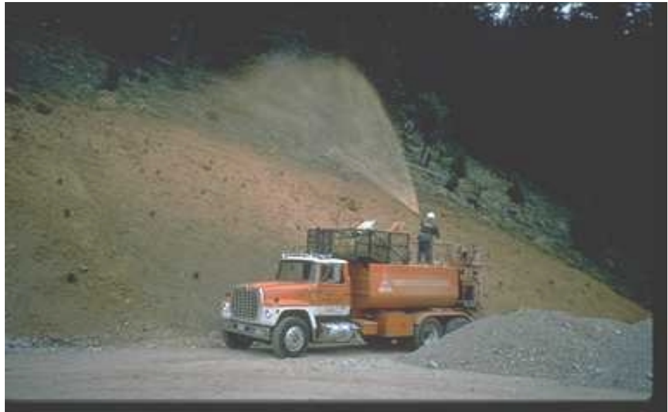
Applying hydraulic mulch.
